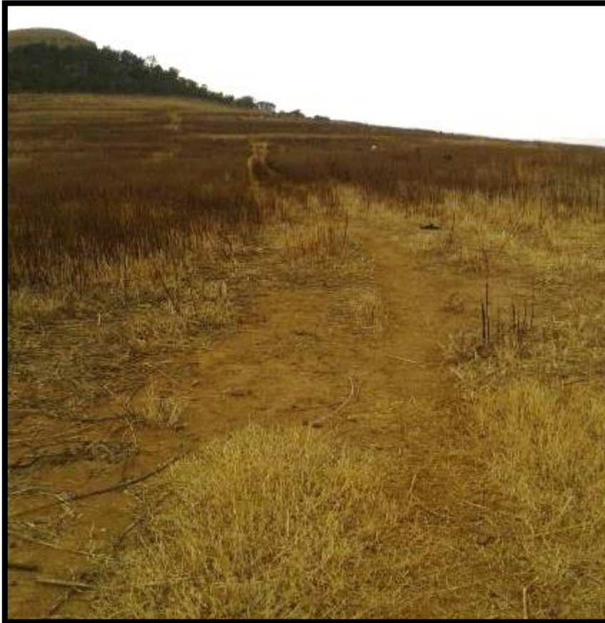
Figure 3. The proposed road upgrade follows an existing track. No heritage sites occur on the footprint.
