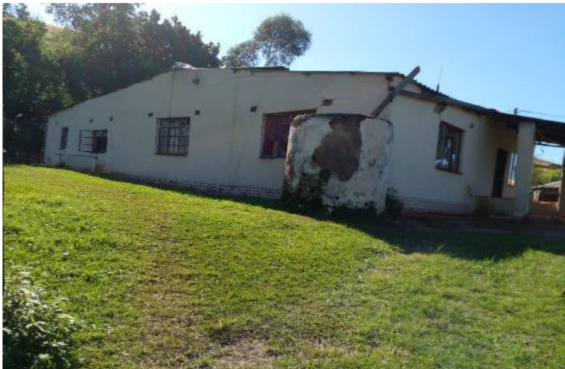
Figure 12: Possible protected structure
