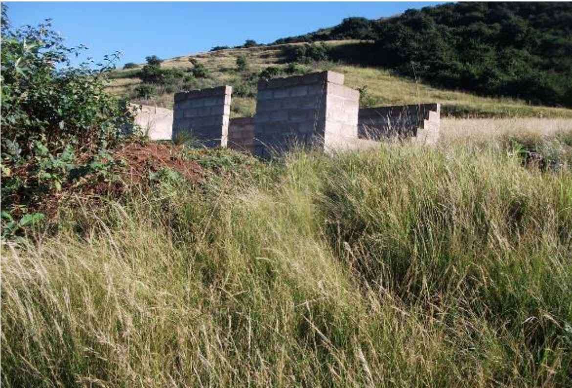
Figure 6: Construction of new structure with project area in background
