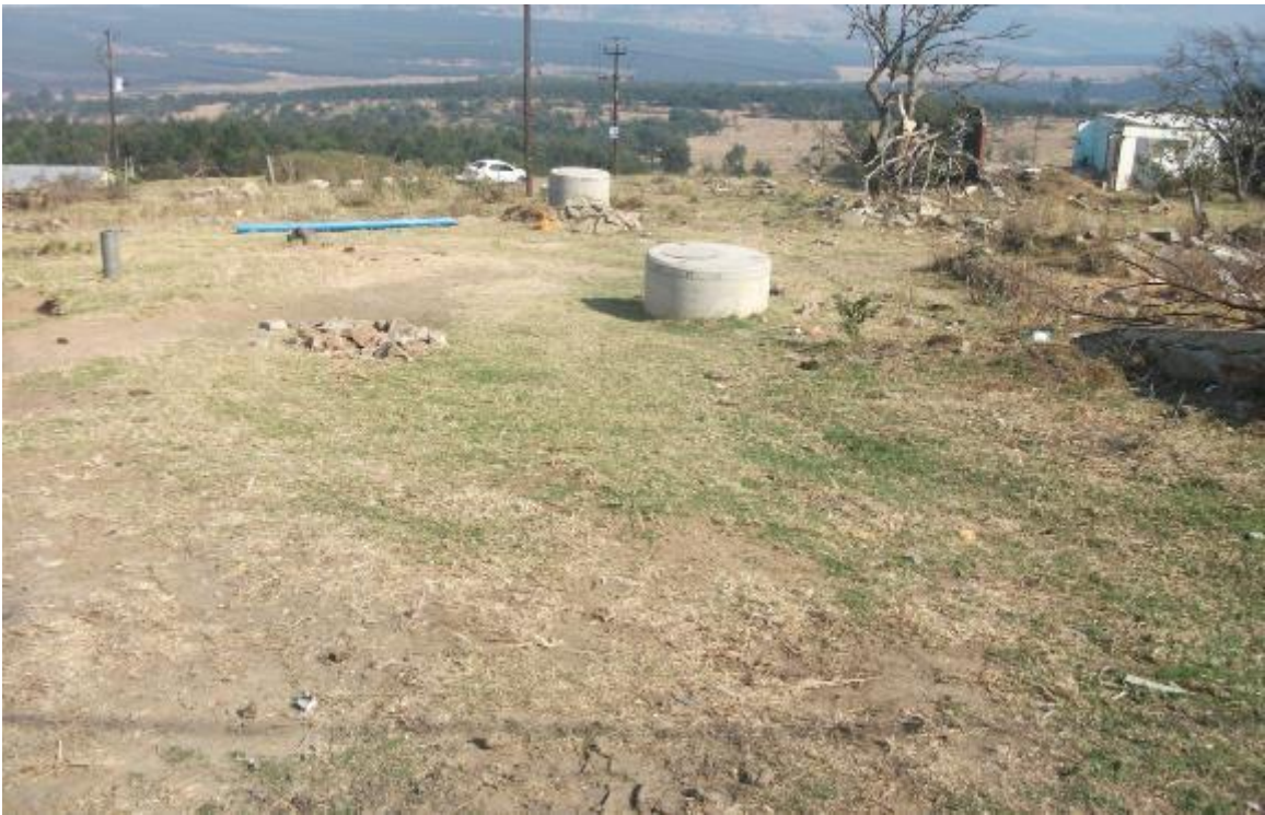
Figure 11: View of pipeline route showing new man-holes
