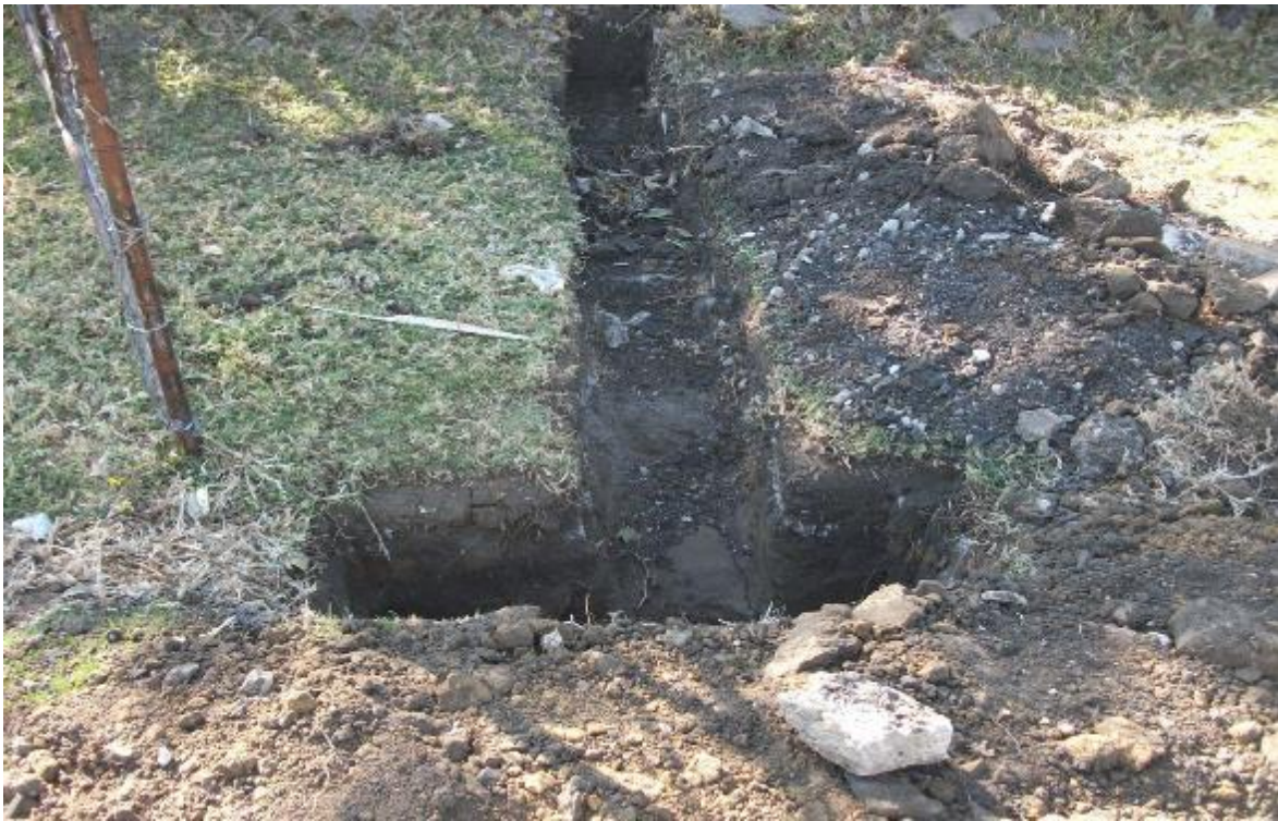
Figure 5: Dug section entering property from road
