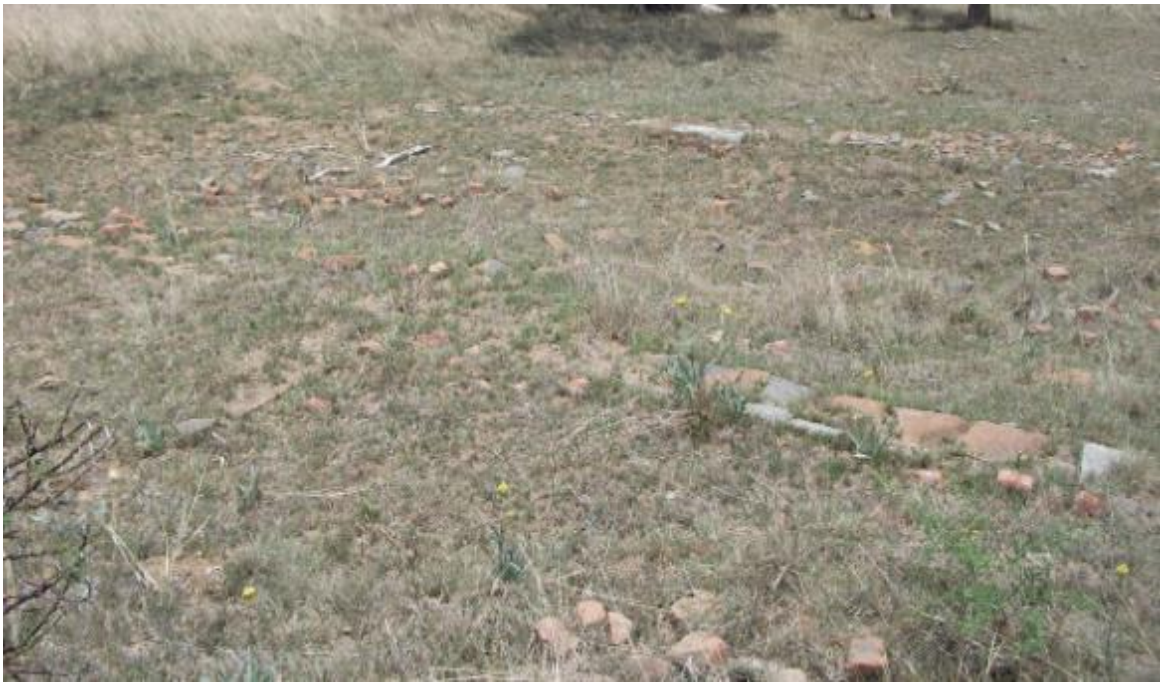
Figure 11: Remains of foundations of walls of structure
