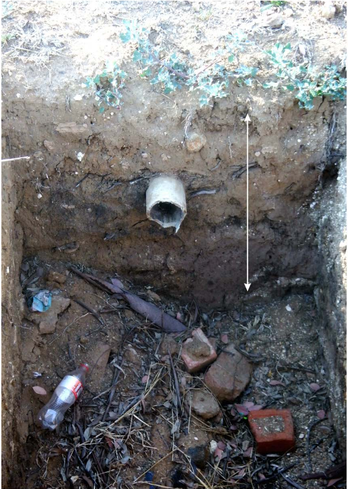
Figure 9. Excavation showing part of a section through the superficial overburden at Plot 146.
