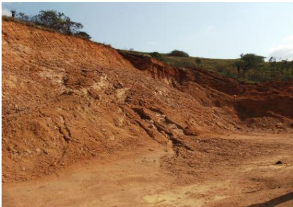
Figure 11: Quarried area of borrow pit
