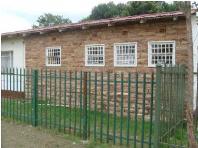
Section of old sandstone structure at School
