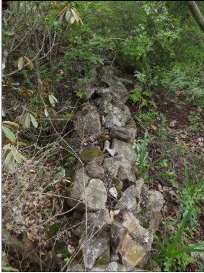
Fig. 6. Site BH 2. The wall is perpendicular to a large waterpipe located a few metres north.
