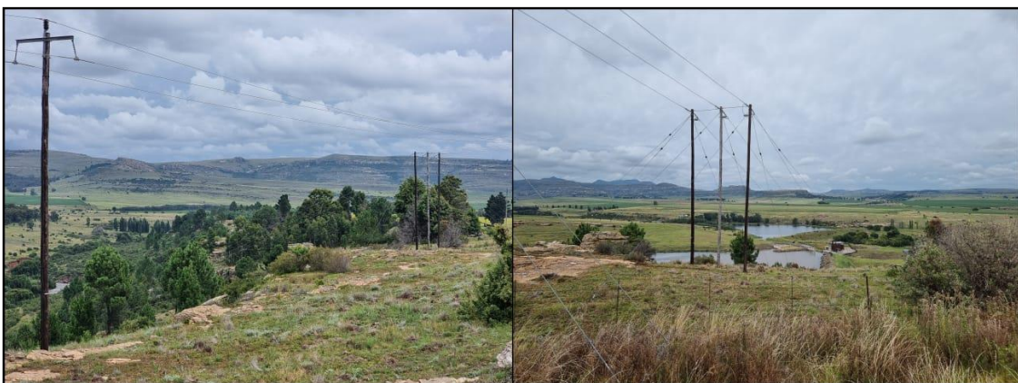
Figure 5-1: View of existing ESKOM power lines in the project area.
