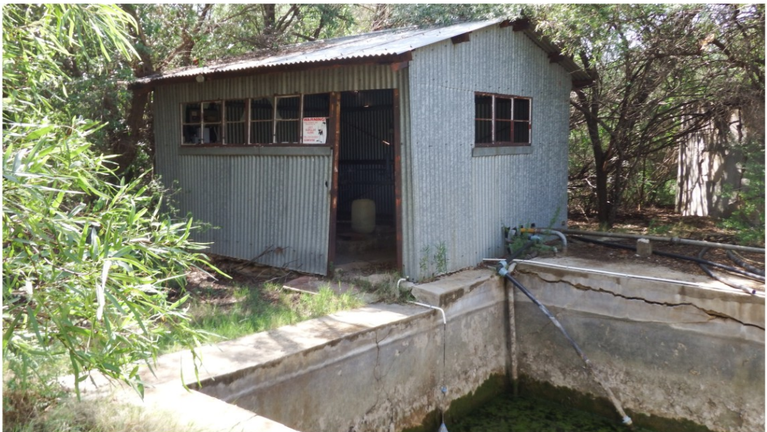
Figure 18 . Dam wall and pump house at GPS 157 (marked no. 6 in Fig. 13).
