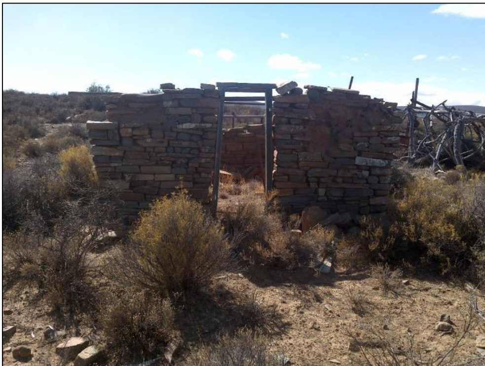
Figure 38: Close-up view of the stone walling cottage (BV_SW4) facing east.
