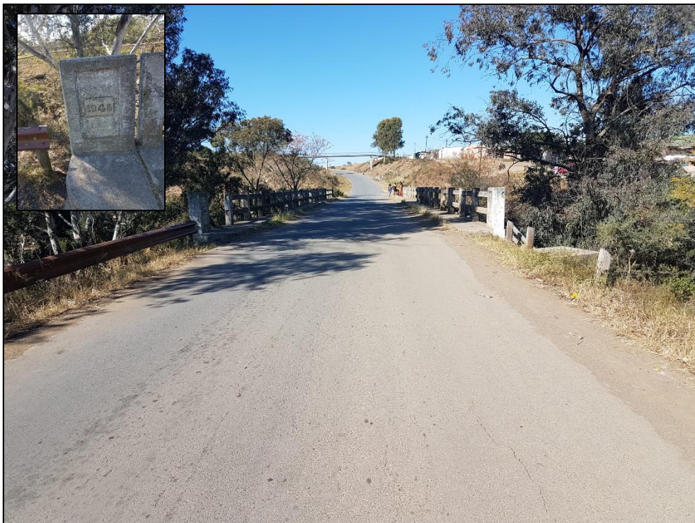
Figure 23. View of the bridge along the access road to Acorn Valley built in 1948.
