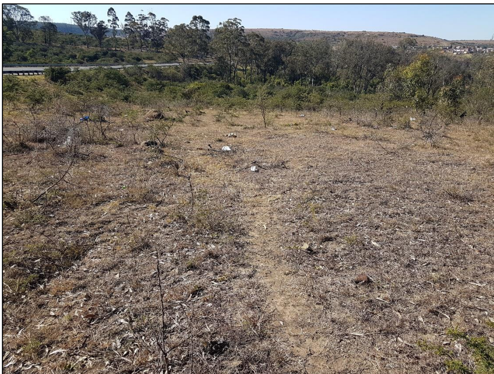
Figure 19. View of the pipeline route along Welkom Road towards Zwelitsha showing the general landscape.
