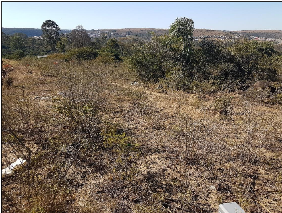
Figure 20. View of the pipeline route along Welkom Road towards Zwelitsha showing the general landscape.
