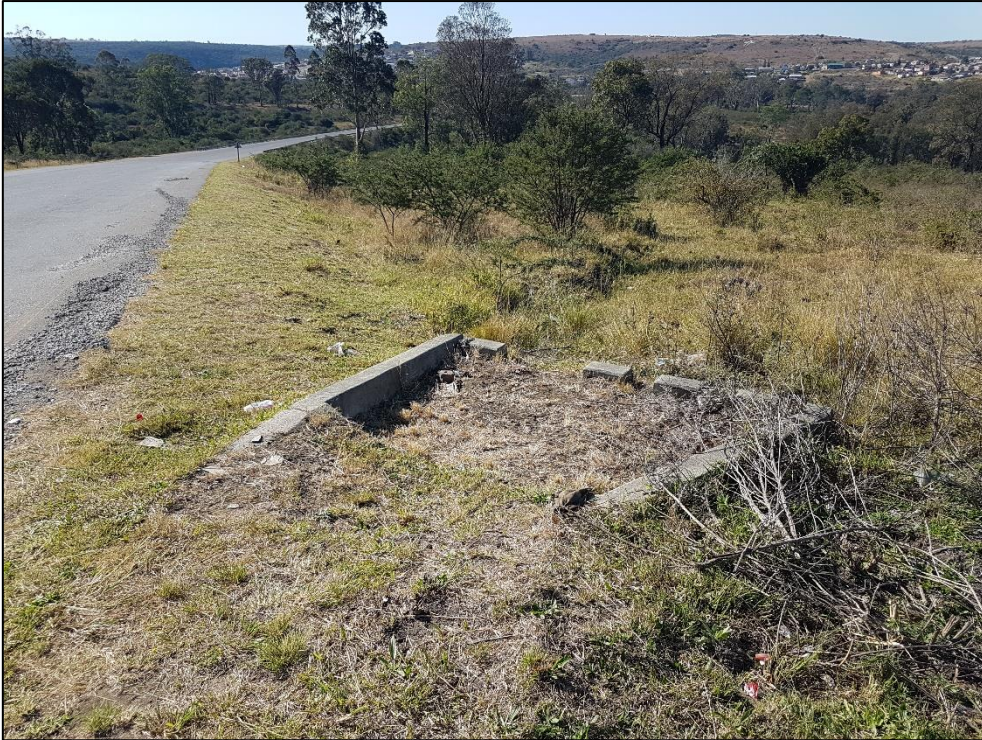
Figure 26. View of a built environment structure along Welkom Road.
