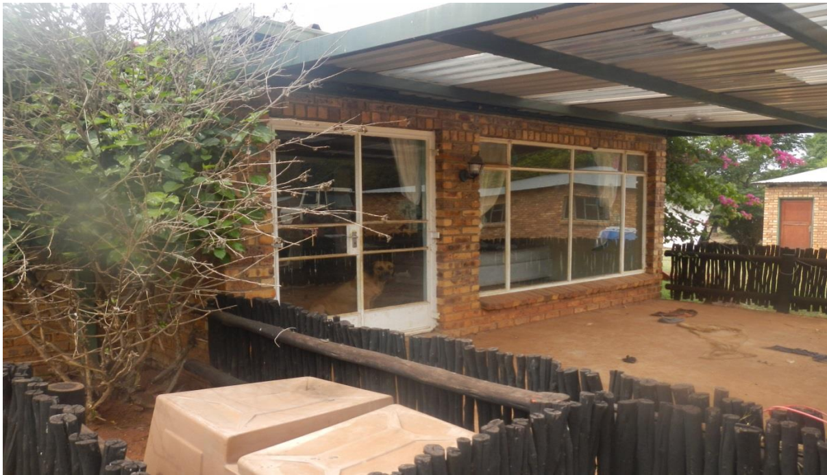
Figure 5: Front end faced of the farm house. Notice the French door and the new windows that serves as proof this building cannot be an old building (60years or older).
