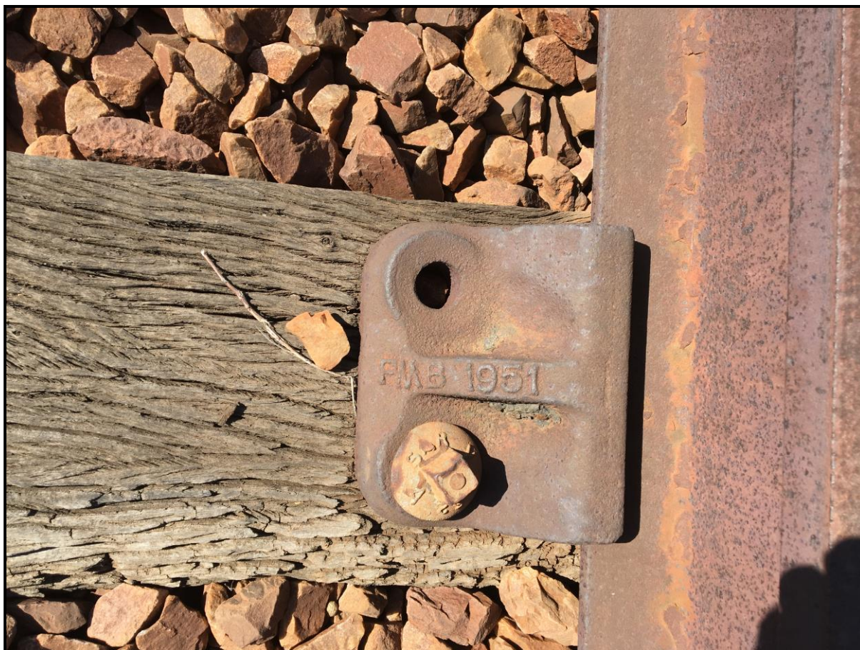
Figure 21: Stamp on the railway indicating an approximate date of 1951 for the railway lines.
