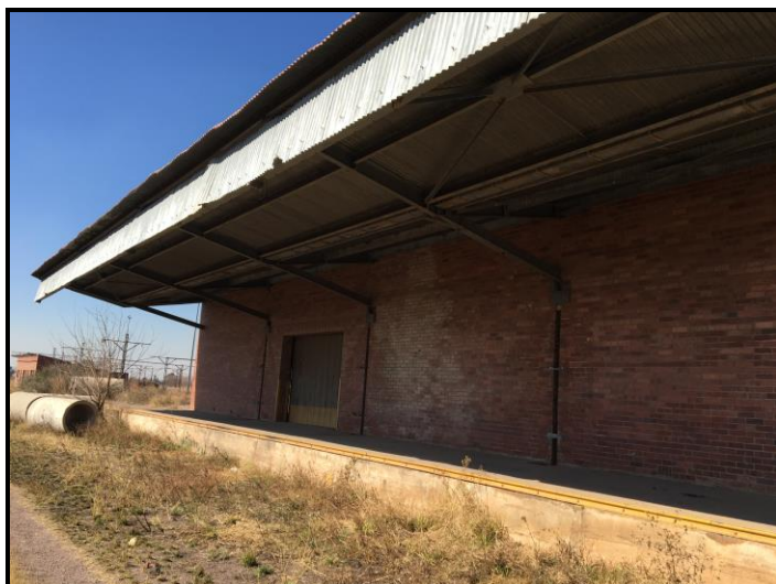
Figure 22. Large storage space.
