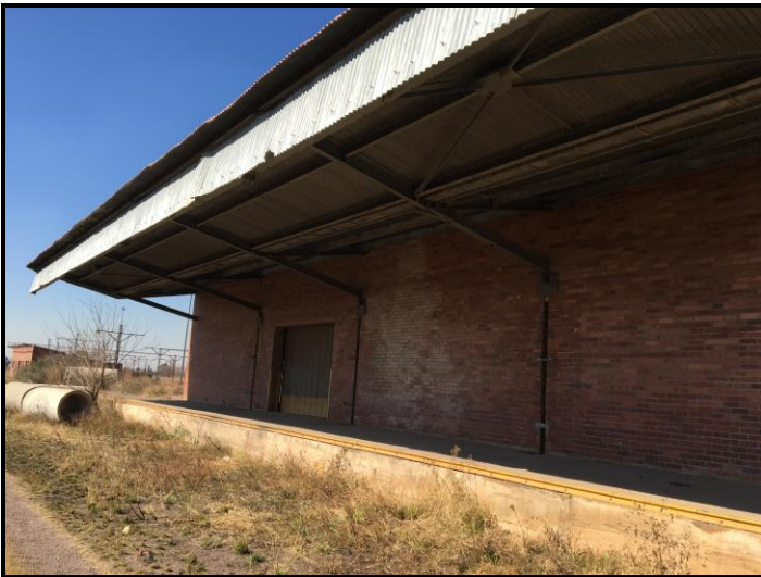
Figure 22. Large storage space.
