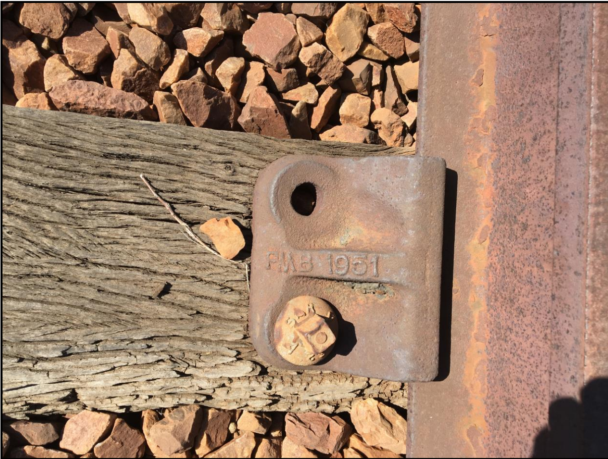
Figure 21: Stamp on the railway indicating an approximate date of 1951 for the railway lines.
