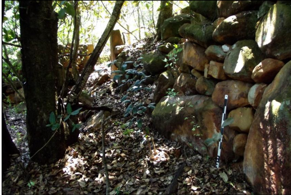
Fig. 21. Site BL 4B. A similar photo as fig. 20. Showing the entrance and height of the walls is indicated with the photo scale in the foreground.
