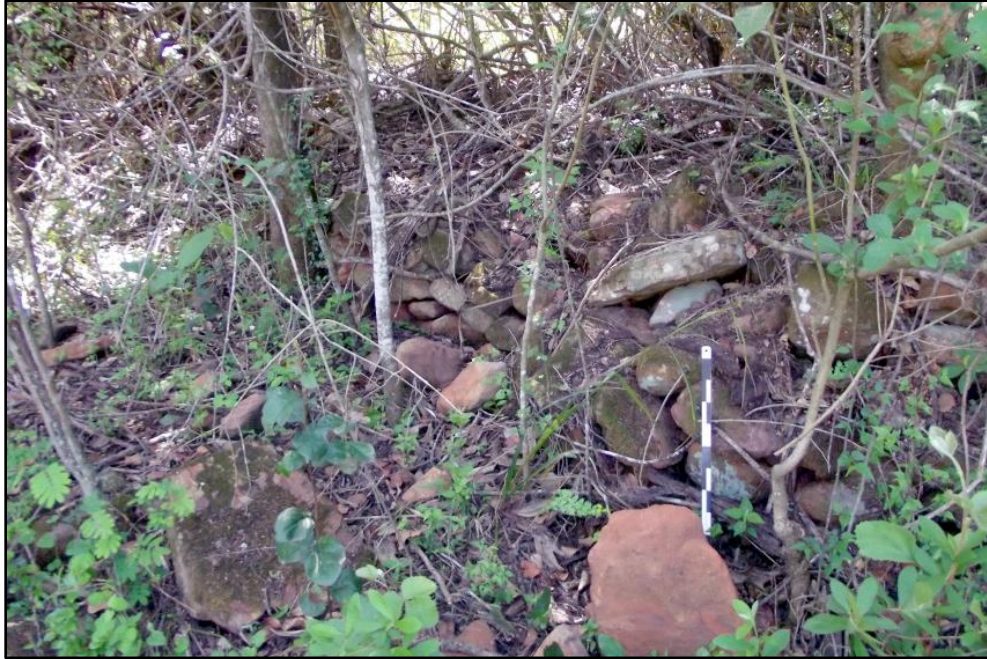
Fig. 15. Site BL 3. Collapsed stone-walling of a LIA stone-walled enclosure. Photo taken in a north western direction. Scale is 0,5m.
