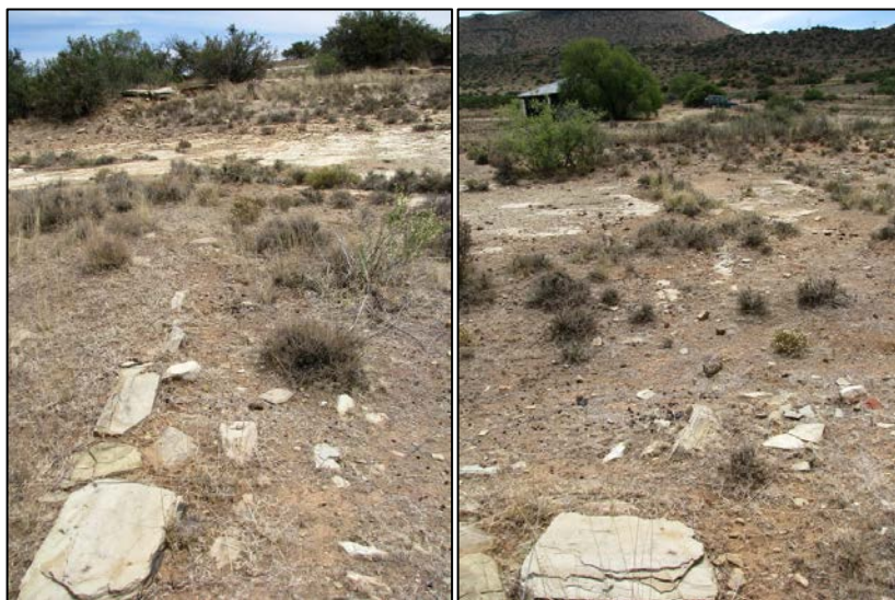
Figures 25 & 26: Foundation of unidentified structure.
