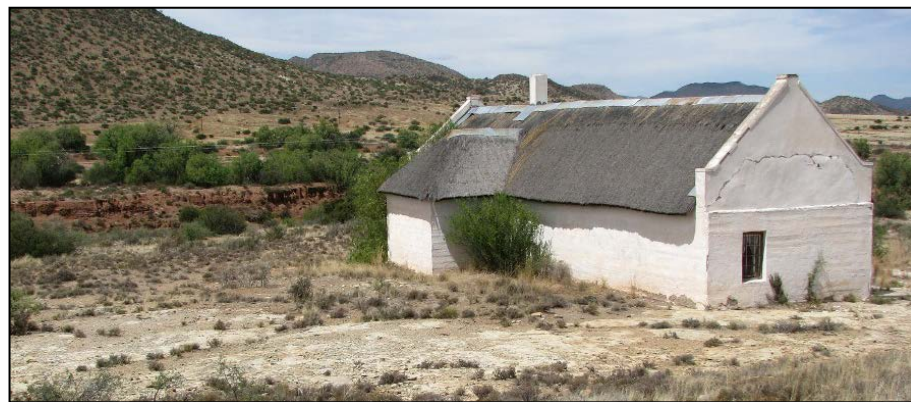
Figure 24: Rear view of house where foundations are still visible.
