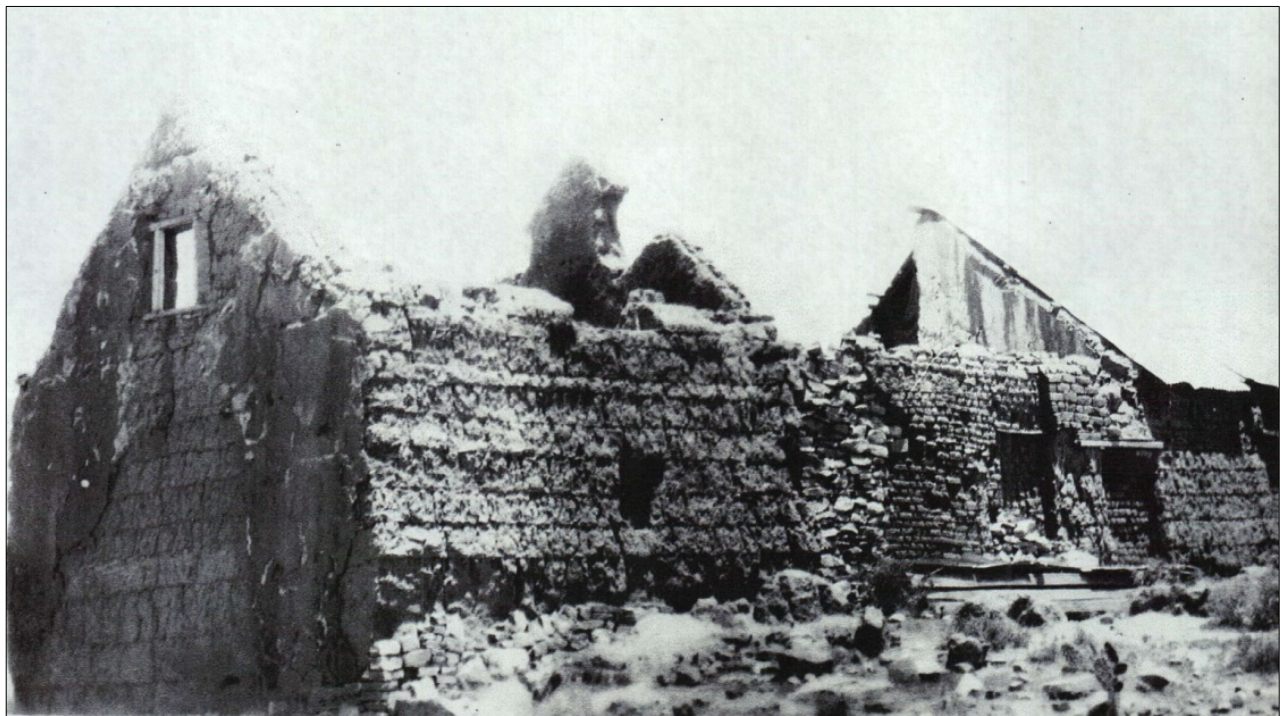
Figure 10: The remains of the main house after it was damaged in a fire.
