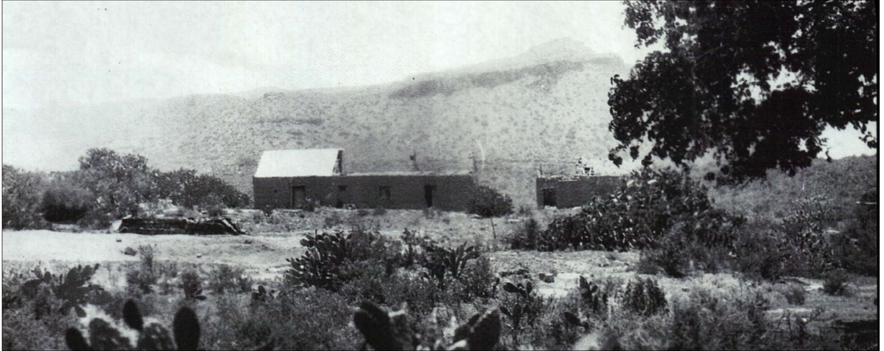
Figure 11: The remains of the main house, as well as those of a house next to it, after it was damaged by a fire.
