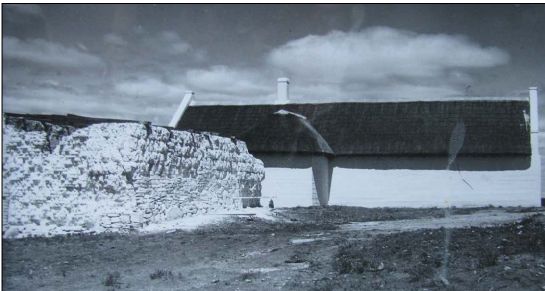
Figure 21: Unidentified structure behind house, 1938.
