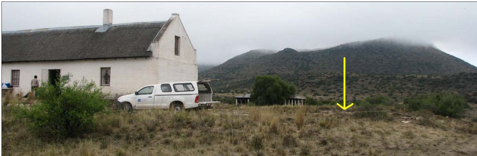
Figure 13: A recent photo of the main house at Bulhoek, indicating where the other house once stood.
