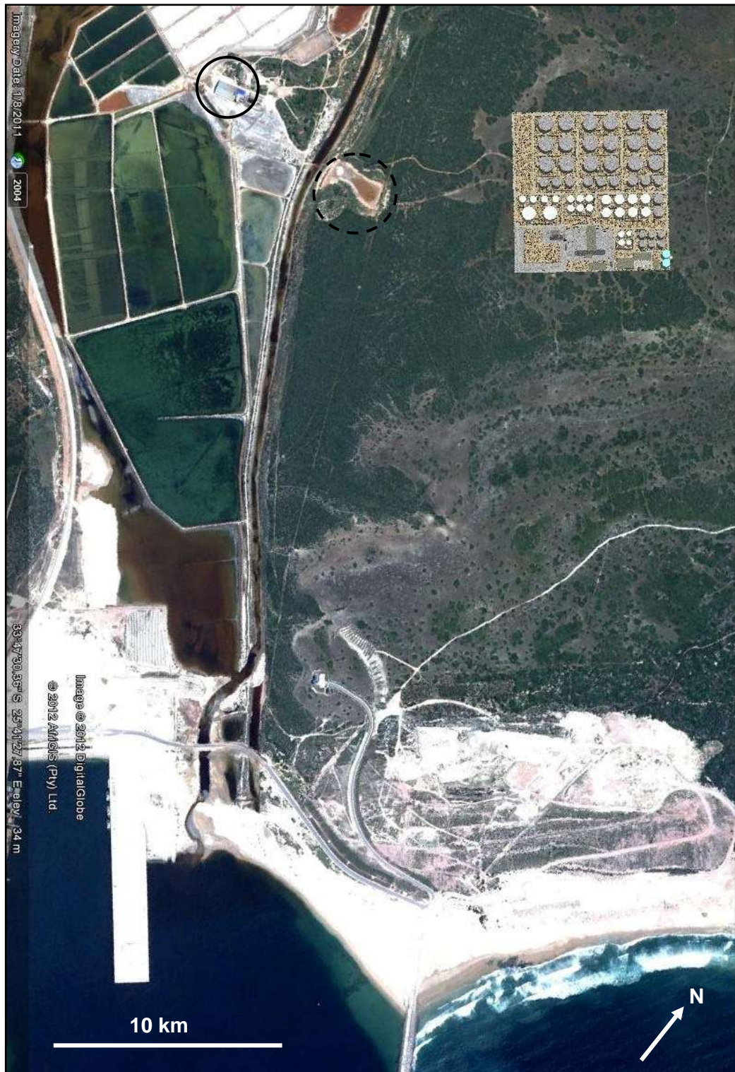
Figure 14.3: Google Earth® satellite image of the OTGC tank farm study area (brown square) on the eastern side of the Coega River. The solid black circle shows the Stratotope D section of the Salnova Formation west of the Coega River. The dashed black circle indicated good exposures of fossiliferous Salnova sediments on the eastern bank of the estuary. Compare with Figure 14.2 for location of pipeline routes to existing or future berths in the port area.
