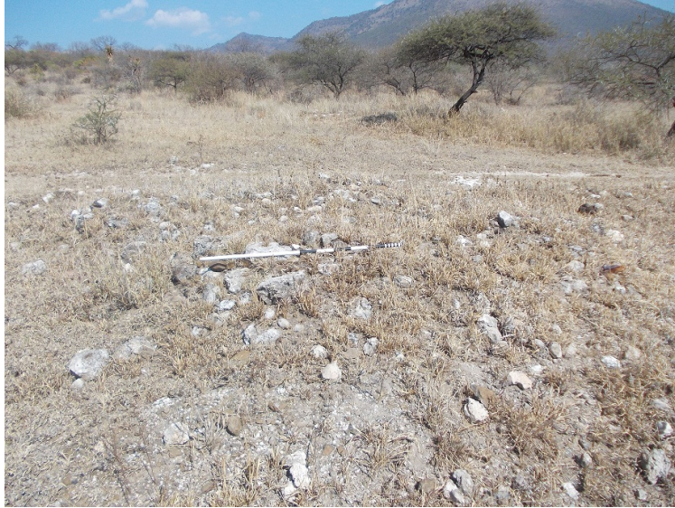
Fig 1. View of historical foundation
