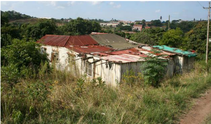
Fig 1: Wood-and-iron structure from the rear.
