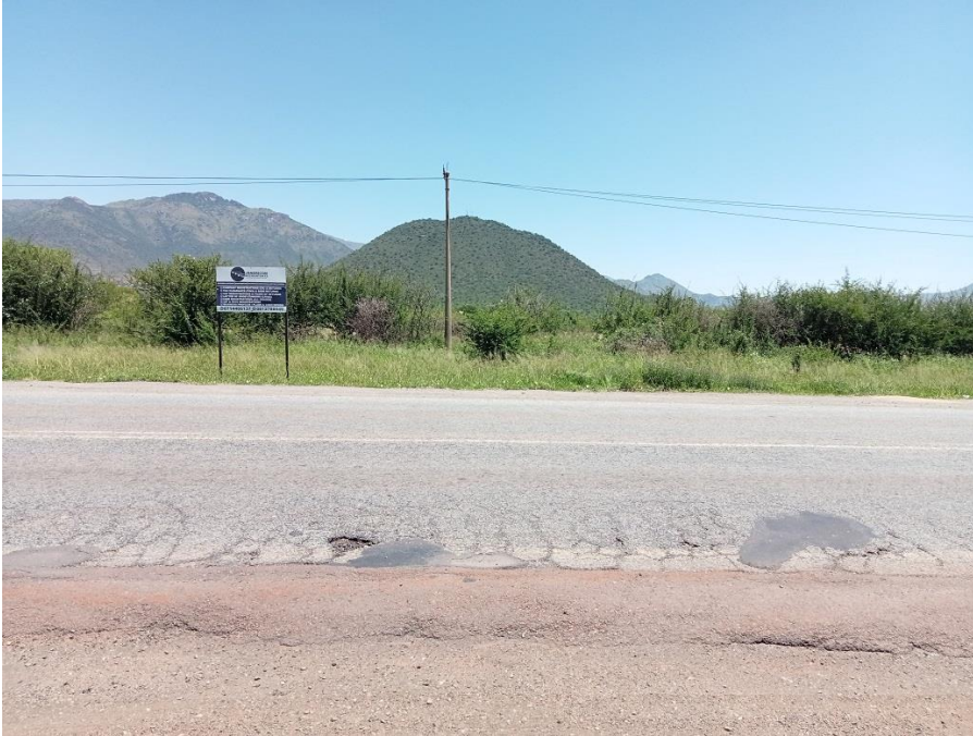
Figure 10: View of R555 where the deviated powerline intersects the road on the western side.
