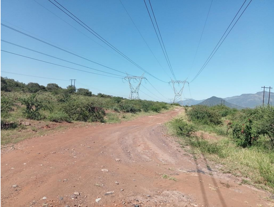
Figure 6: View of existing powerline along the deviation.
