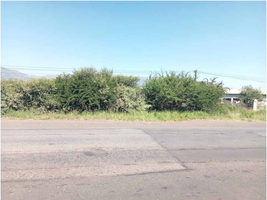
Figure 9: View of R555 where the deviated powerline intersects the road on the eastern side.
