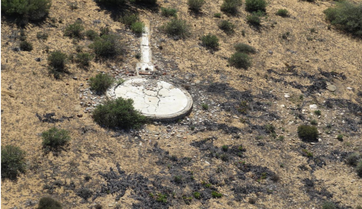
Figure 14: View of an abandoned structure.
