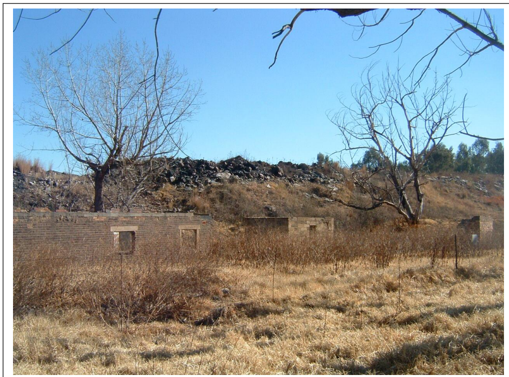
Figure 7- A historical residence (S01) with outbuildings on Haverklip 269IR. These structures were constructed with face bricks and cement and are partially still intact (above).
