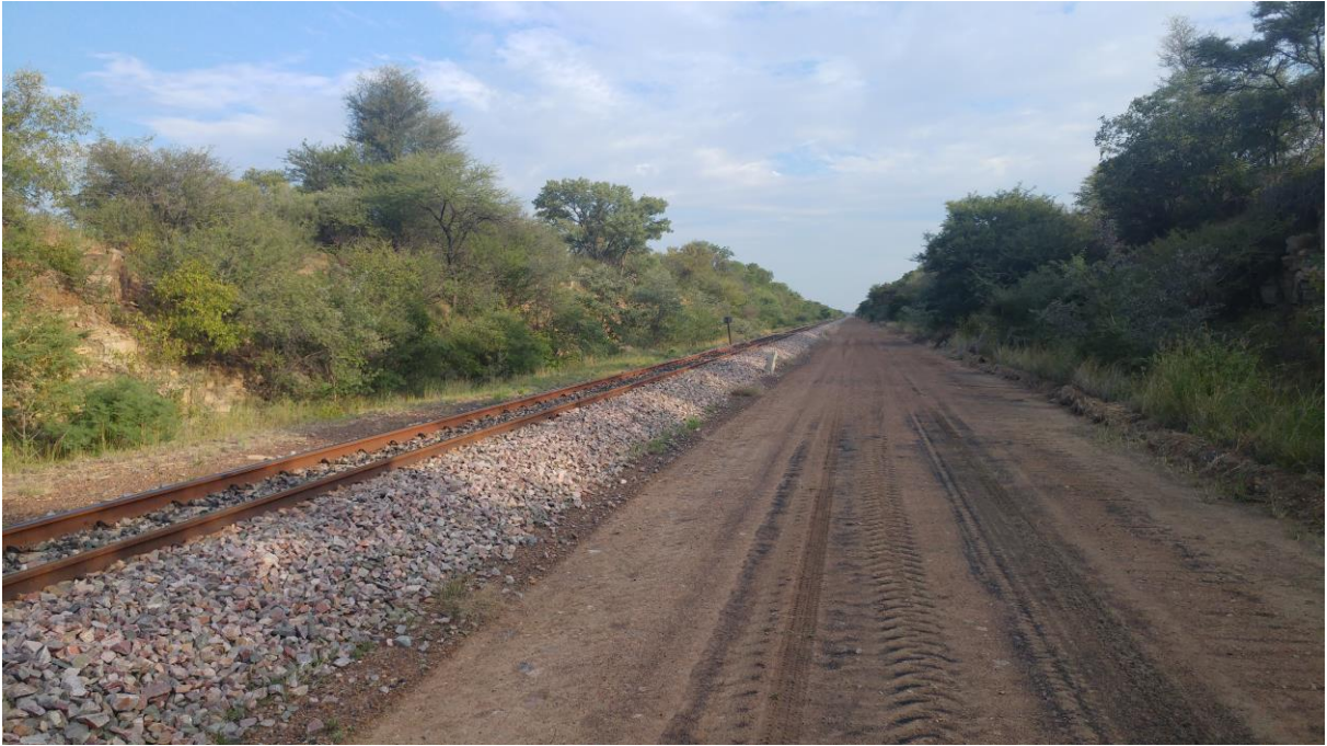
Figure 16: General view at the proposed site for the substation.
