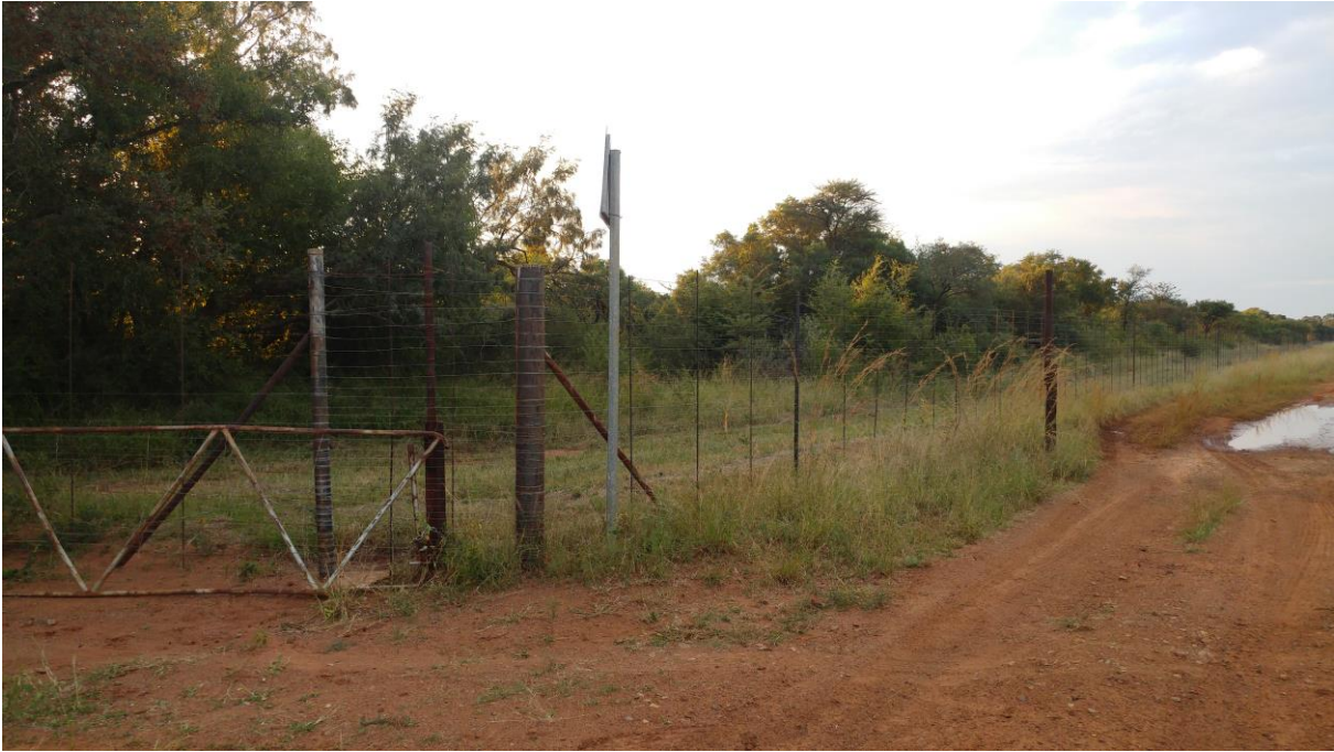
Figure 14: General view at alternative 1 for the substation.
