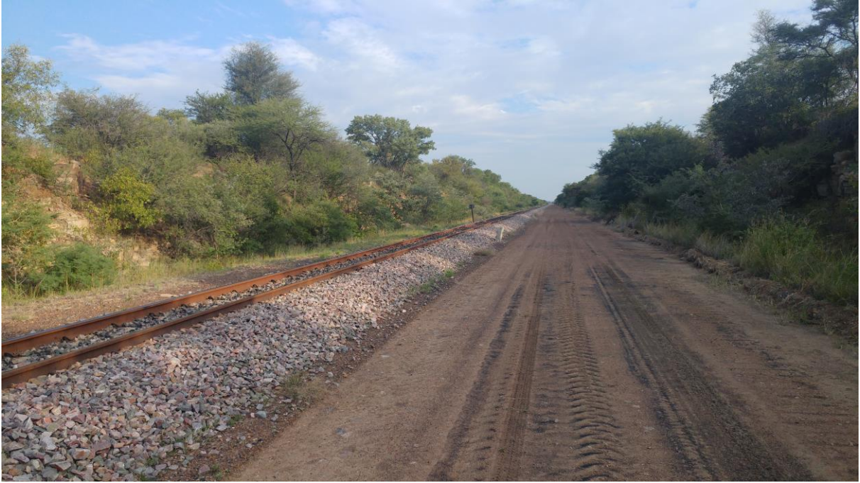
Figure 18: General view at the proposed site for the substation.
