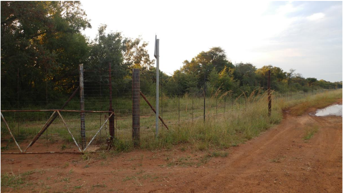
Figure 16: General view at alternative 1 for the substation.
