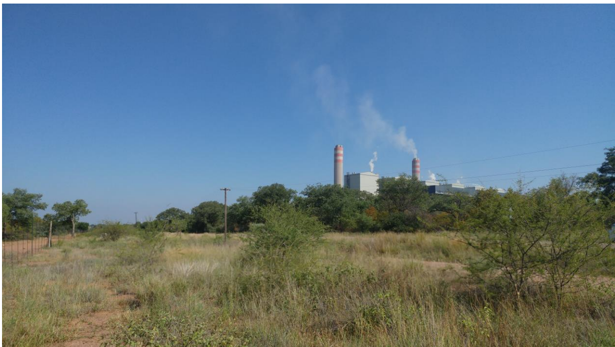
Figure 23: General view of the surveyed area close to the Medupi Power Station.
