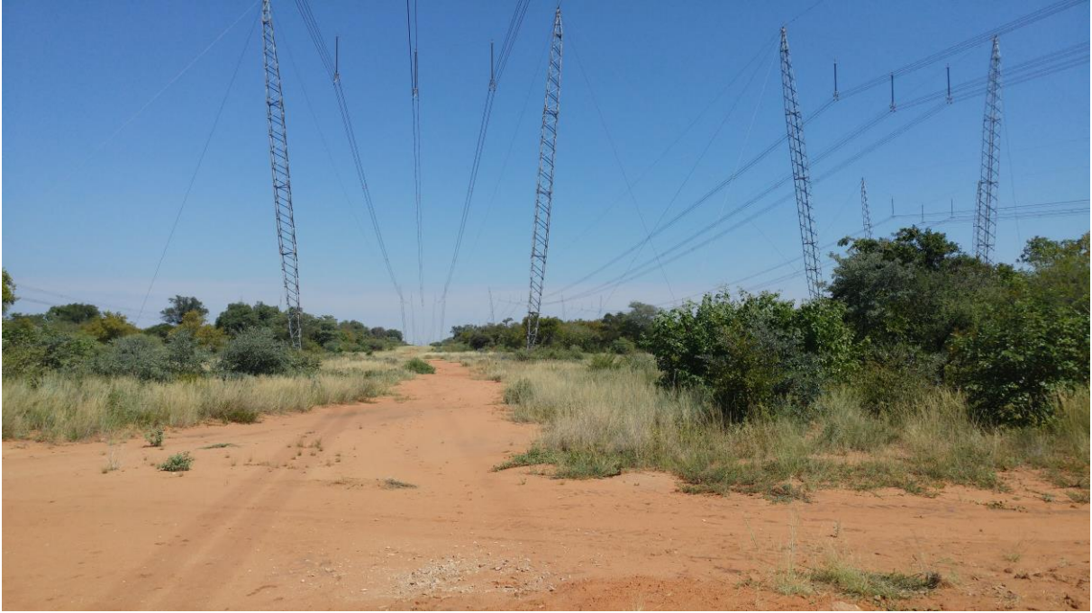
Figure 26: Existing power lines along the proposed routes.
