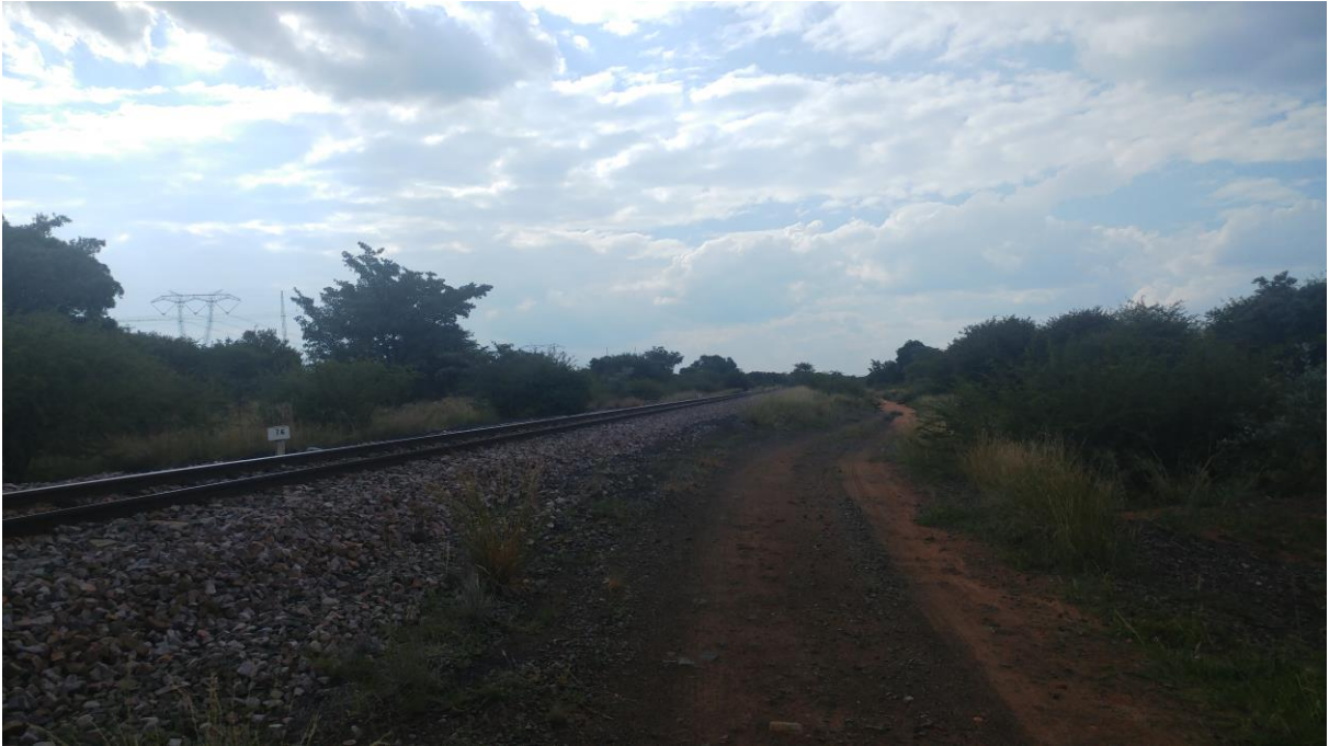
Figure 22: Another view at the proposed substation site.
