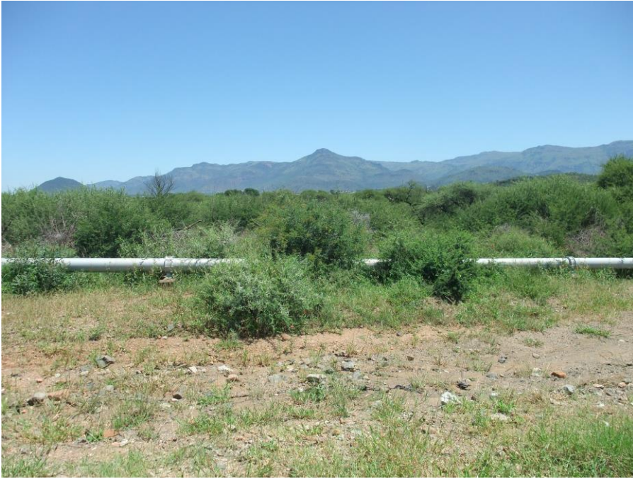
Figure 11: Industrial pipe line along the route.
