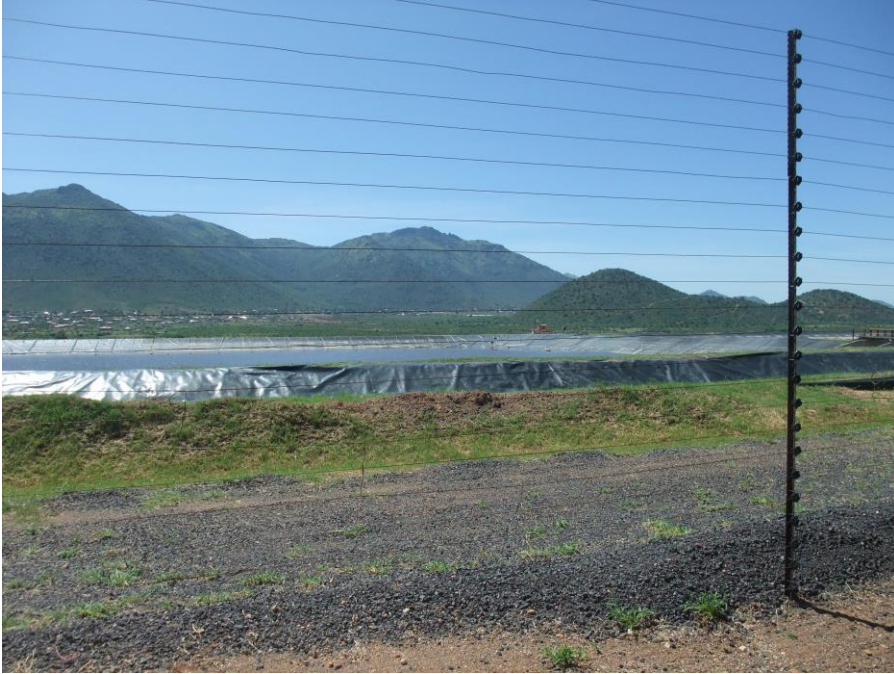
Figure 13: Dam within the corridor.
