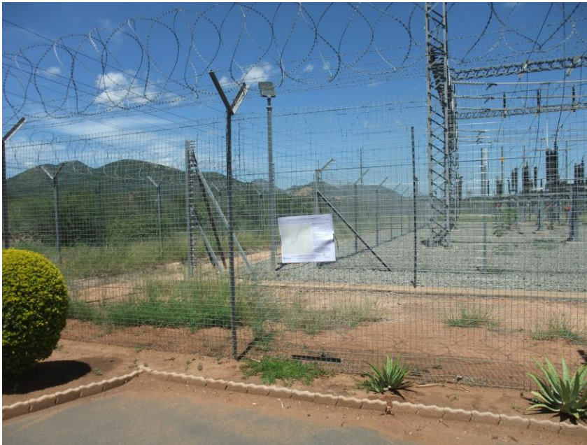
Example of site notices – this one at the Merensky substation.
