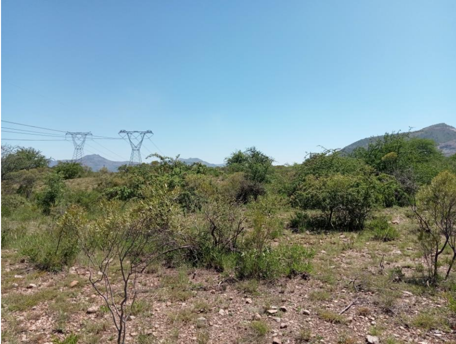
Figure 7: View of vegetation growth between points E and G of the deviation.
