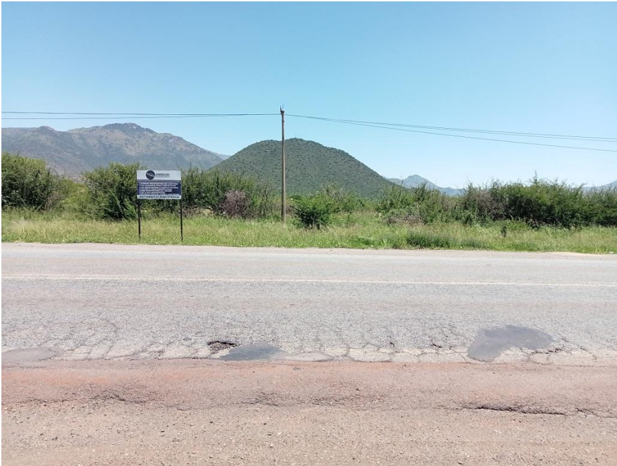
Figure 10: View of road where the deviated powerline crosses, between points F and G.
