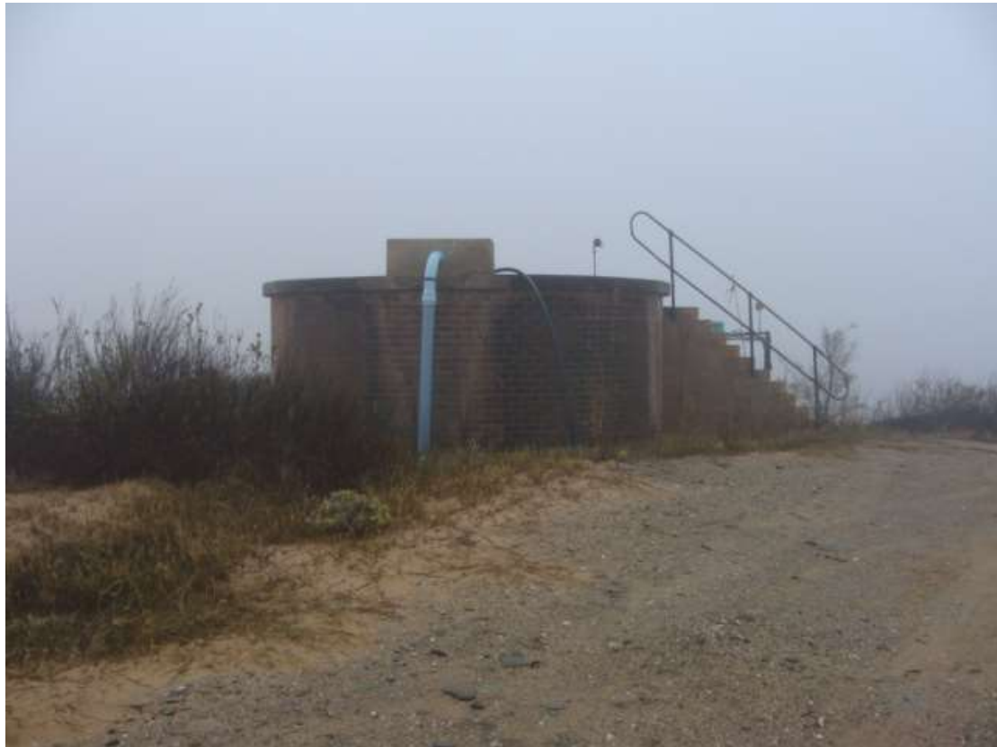
Figure 17: Reservoir on the above mentioned hill.
