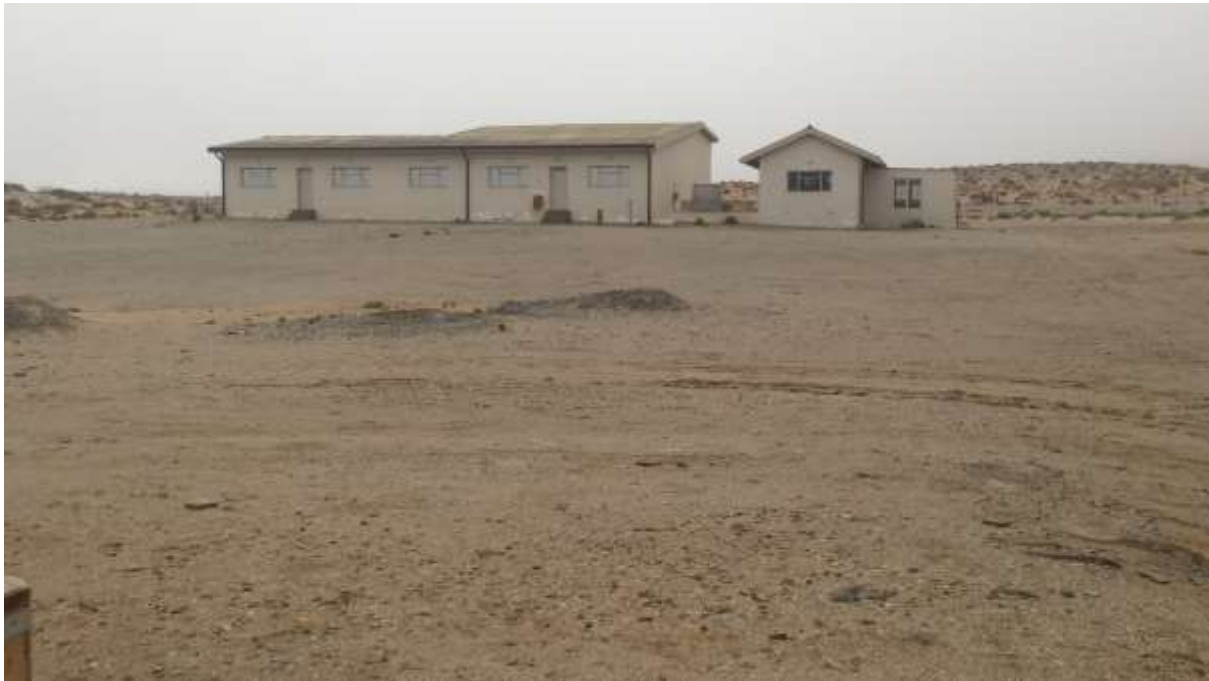
Figure 15: Some of the buildings at the substation that will be demolished. None of these are older than 60 years and has no heritage significance.
