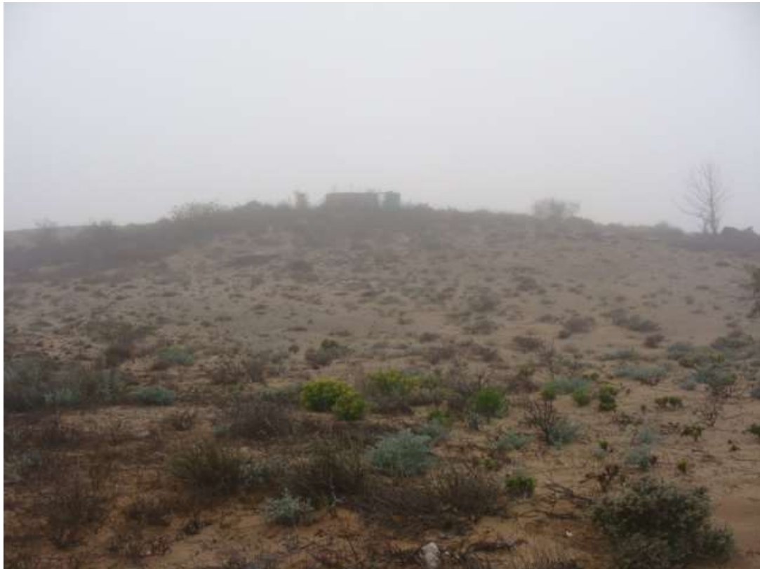
Figure 16: Hill adjacent to the substation showing signs of disturbance.
