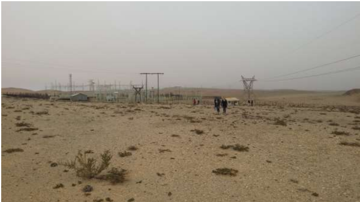
Figure 18: View along the current substation.
