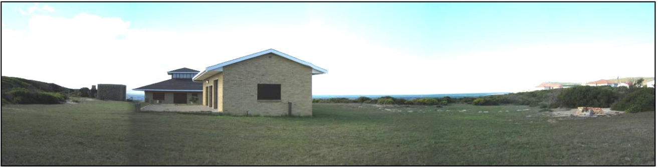
Plate 1: Existing structures on the northern part of the site showing the landscaping.
