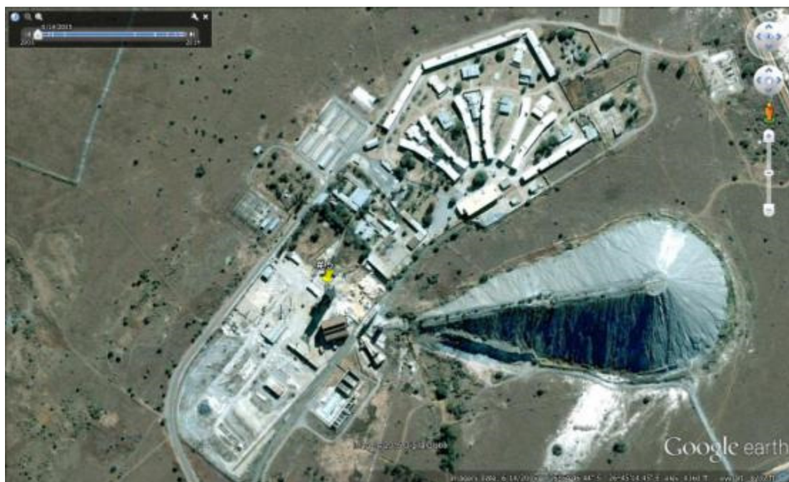
Fig. 53. Above is the site map of the #5 shaft and its associated infrastructure. (Google Earth image 2005.) From this image it is clear that portions of the site are still intact although demolition has already commenced. 15 Compare to figure 50 dated 2014.
