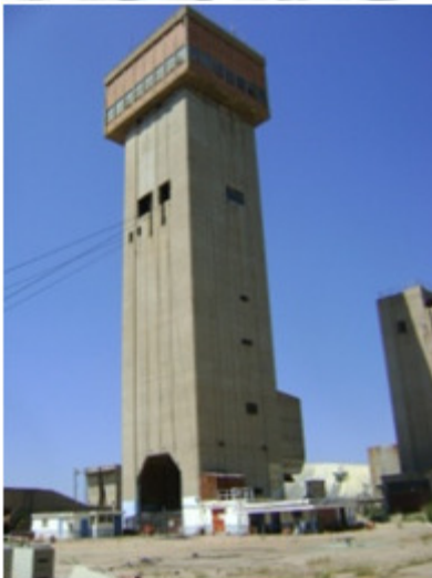
Fig. 30. Left is the concrete headgear structure of #2 shaft. The presence of a concrete headgear such as this one normally indicates modern technology and origin period post 1950 8 . (Photograph, S.M. Miller 2015.)
