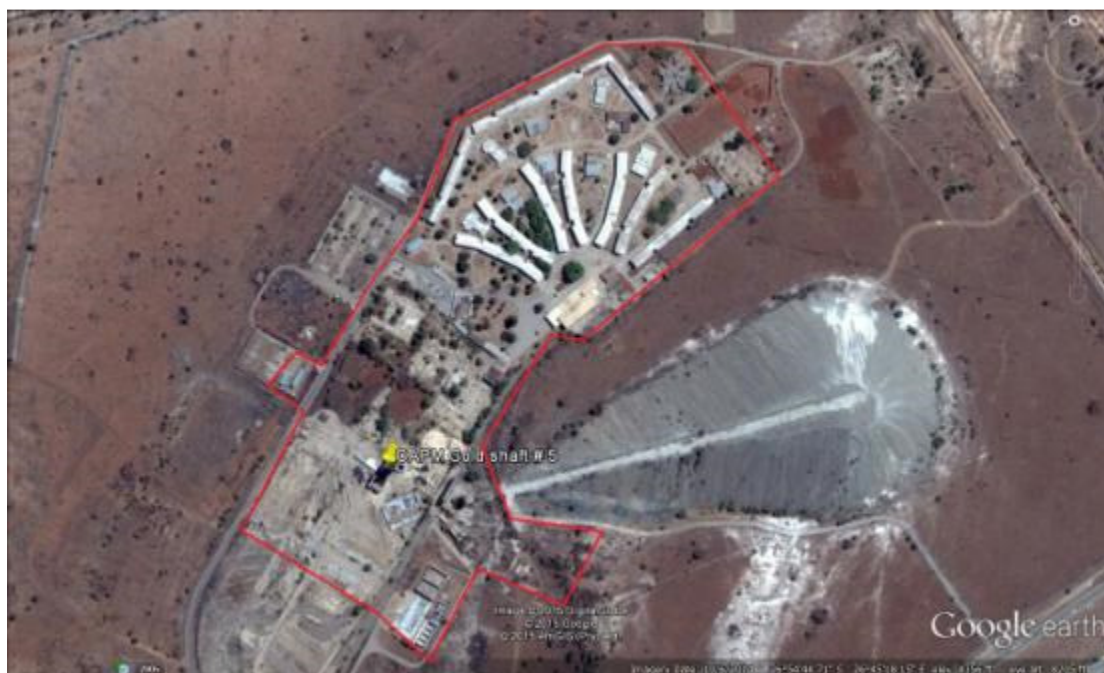
Fig. 50. Above is the site map of the #5 shaft and its associated infrastructure. (Google Earth image (2014) and the investigation area is outlined in red.)(For full list of official buildings and infrastructure see appendix in the 2015 E.I.A complied by Shangoni Management Services.)
