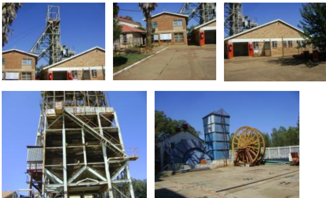
Figs. 57 to 61. Above are typical buildings and structures on site of #6 shaft. All date from circa 1940 and onwards. The entire infrastructure on this site is to be retained and re-used. (Photographs, S.M. Miller 2015.) 16
