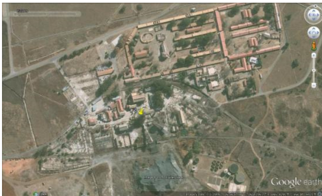
Fig. 43. Above is the site map of the #3 shaft and its associated infrastructure. (Google Earth image 2011.) From this image it is clear that the site is still intact. Note that a large portion of the compound visible here is absent in figure 32 . From the information in figures 32, 42 and 43 it appears that the demolition took place between 2011 and 2015. 12
