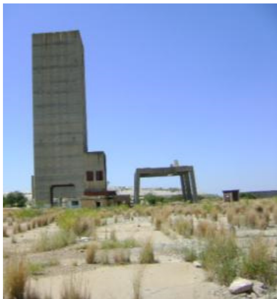
Fig. 52. Left is the concrete headgear structure of #5 shaft. The presence of a concrete headgear such as this one normally indicates modern technology and origin period post 1950 8 . Apart from this lone structure nothing remains from the original infrastructure of the site. (Photograph, S.M. Miller 2015.)
