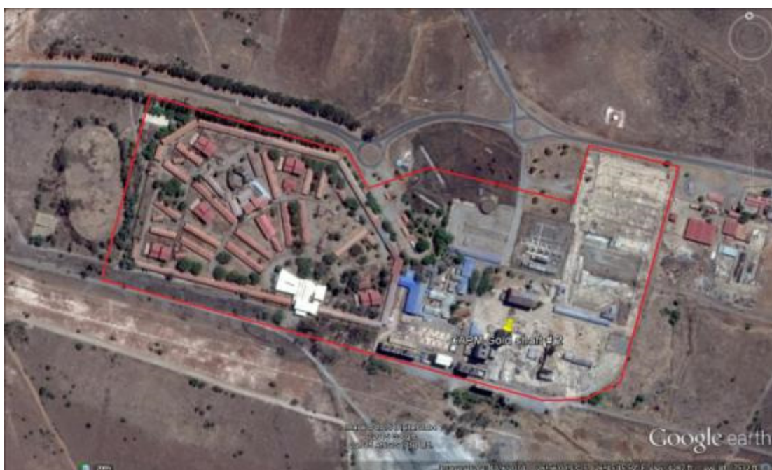
Fig. 24. Above is the site map of the #2 shaft and its associated infrastructure. (Google Earth image (2014) with the investigation area outlined in red. 9 )
