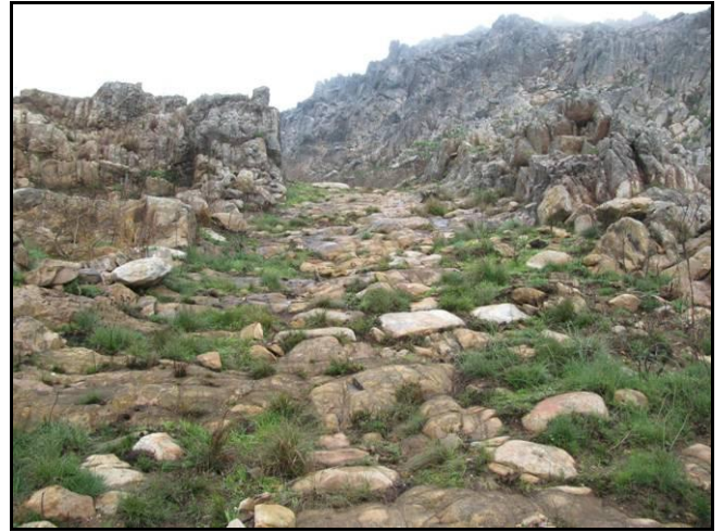
Figure 38: View of the cutting through the sandstone on the upper part of the pass. This is the steepest section.
