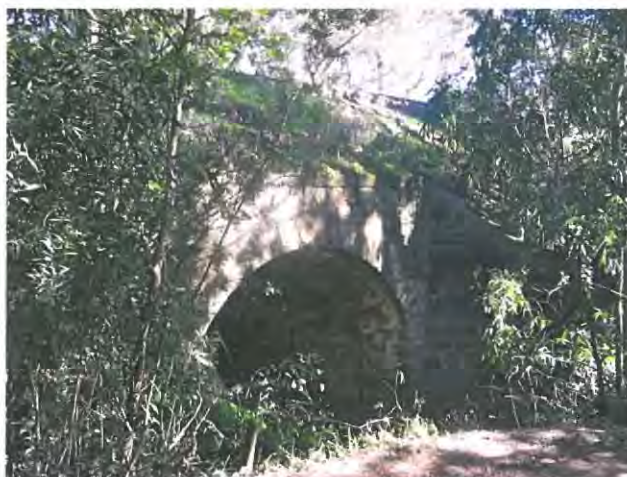
Fig 9. The dressed stone rail bridge c 1901
