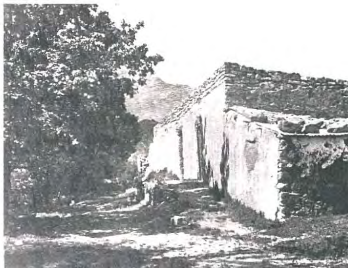
Fig 18. An early photograph (nd) of the Toll house: From P Heap The Story of Hottentots Holland. This shows the building in a ruinous condition. It had a flat roof and the parapet wall levels have been raised. The lean-to, the high stoep, steps, and the door apertures are substantially the same although the stoep is now considerably deeper.
