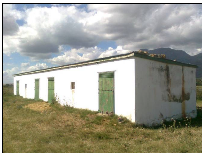
Figure 51: South end of stable.
