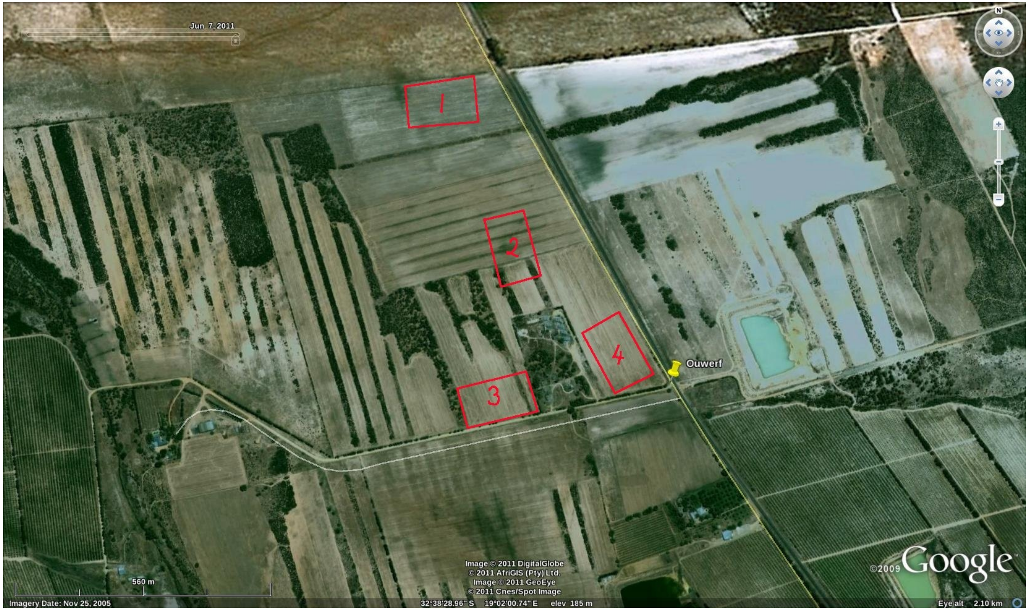
Figure 1: Layout of proposed alternative for the Citrus Packaging Facilities on Ouwerf Farm.
