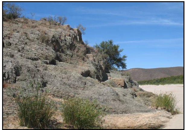
Figure 59: Looking south the some of the footings extending down the rocks.
