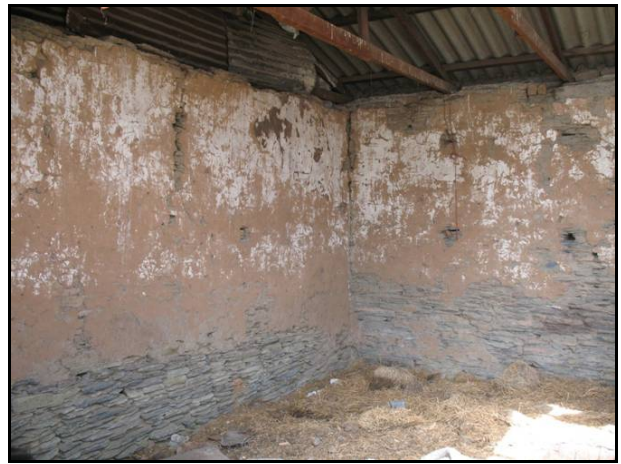
Figure 73: Interior of OD-04.
