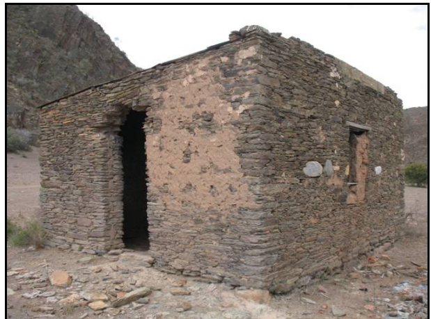
Figure 63: The structure at OD-02.
