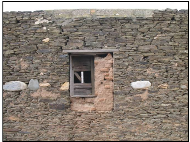
Figure 65: Modified window and parapet at OD-02.
