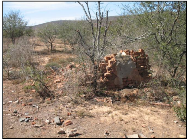
Figure 55: View of second ruined structure at MD-07.
