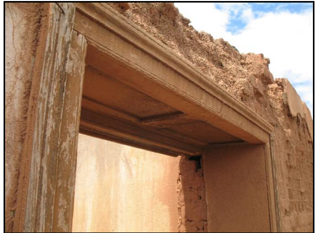
Figure 71: Wood panelling on doorway in OD-03.
