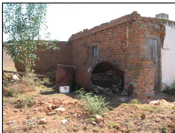
Figure 48: The front left corner of SD-06.
