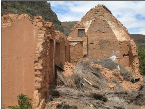
Figure 70: View of the interior of OD-03.
