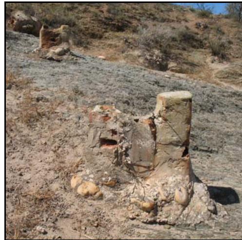
Figure 61: Two footings at SD-08.
