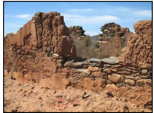
Figure 53: Close-up of the walls at MD-06.
