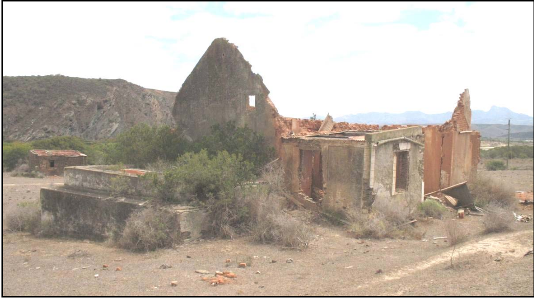
Figure 69: View of the ruin at OD-03 from the southeast. The stone additions can be seen (reservoir at left and extra room at centre).
