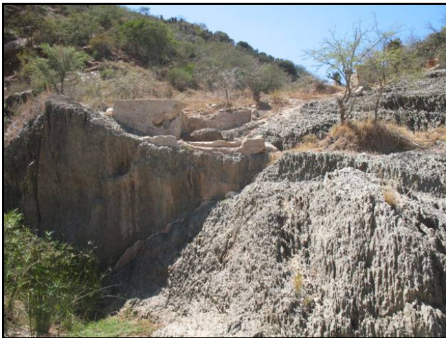
Figure 60: The footings at the base of the stream valley.
