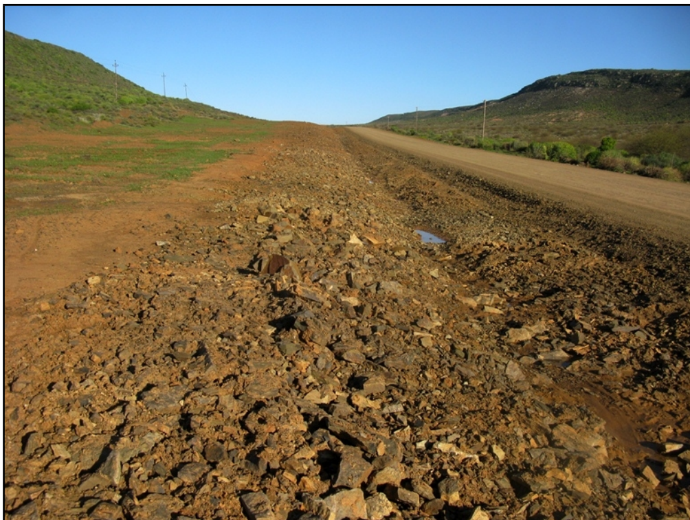
Fig. 10. View SE along the extended roadside borrow pit DR2196/28.5/L/30 (largely rehabilitated). Note lack of bedrock exposure and abundance of ripped-up blocks of Gydo siltstone and wackes.
