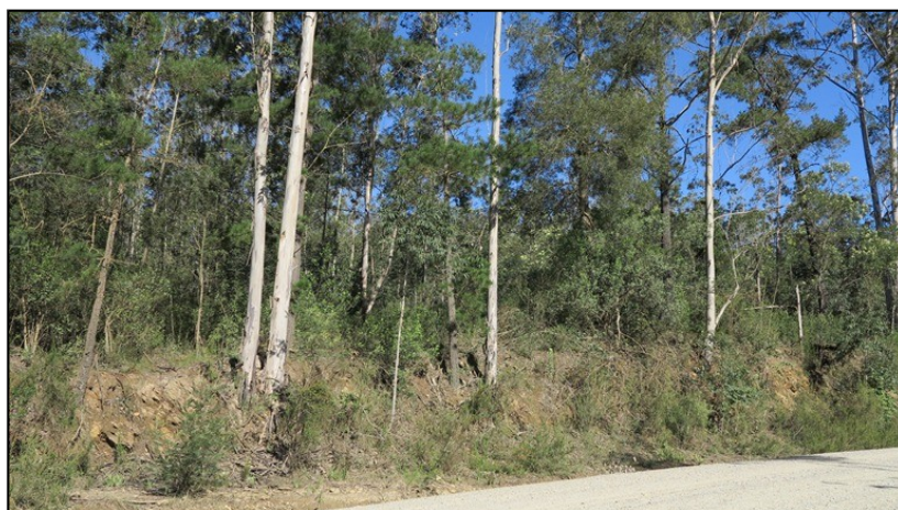
Figure 8: Pit 127 – view towards the southeast with the road cutting along the MR00355 evident below the forested surface.
