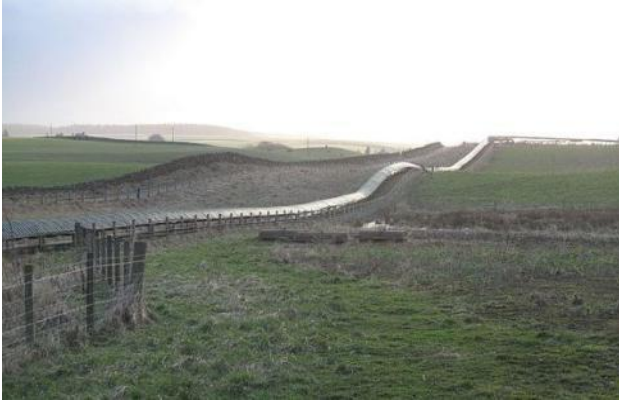
Temple Quarry conveyor ( www.geolocation.com )
