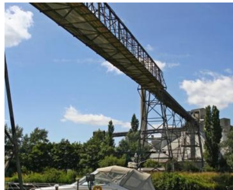
Conveyor Bridge at South Ferriby Marina ( www.geograph.org.uk )
