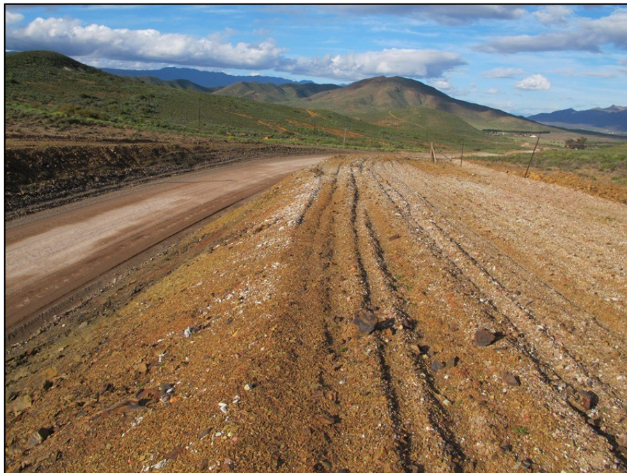
Figure 5: View along the partly-rehabilitated affected area towards the east. The unfenced slope at the eastern end lies beyond the bend in the road.
