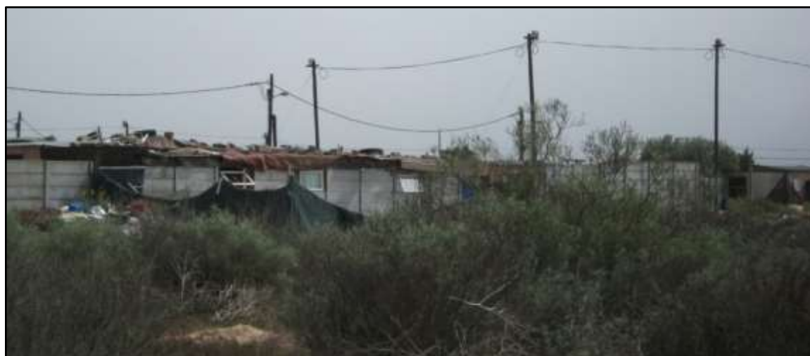
Plate 3: View of the Vibracrete fence toward the north of the existing suburb of Noordhoek showing rubble which has been dumped on the property.
