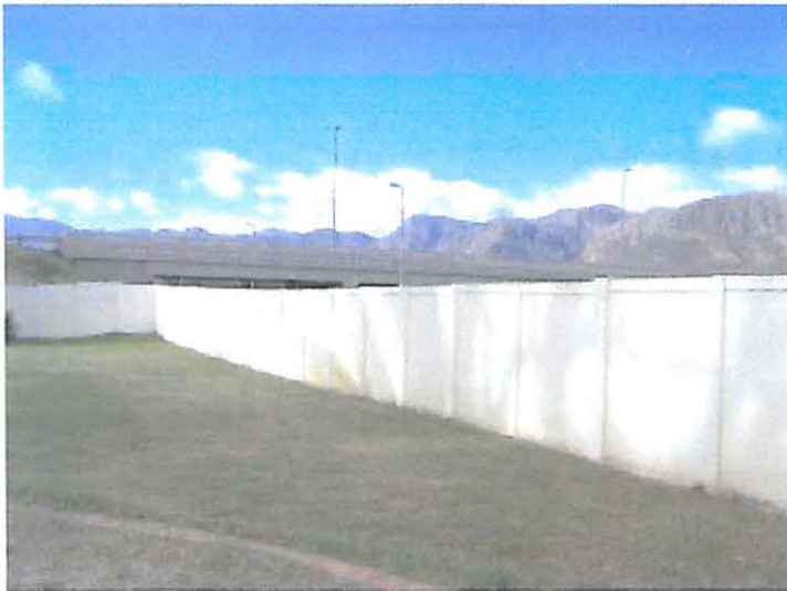
View toward from the property looking toward the Cecelia Road Bridge.
