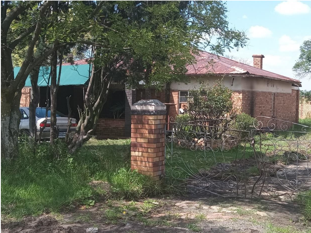
Figure 91: View of the other historical houses
