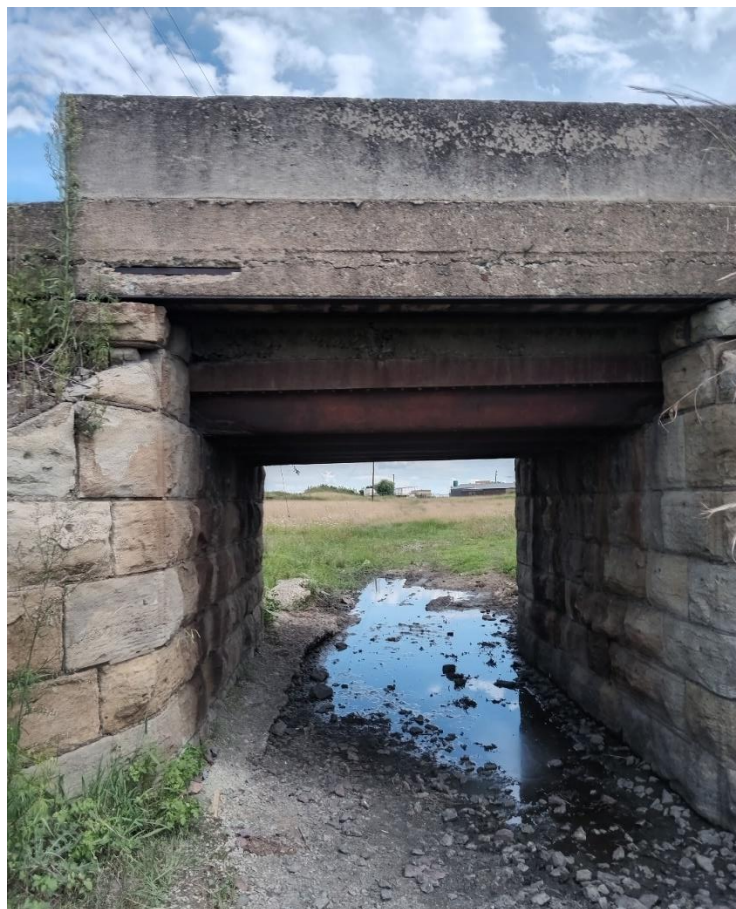
Figure 110: closer view of the stone culvert
