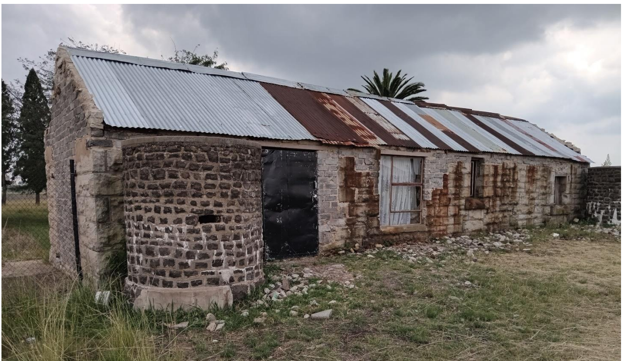
Figure 59: Closer view of the Sandstone outbuilding, showing two circular features next to the west and east ends of the building
