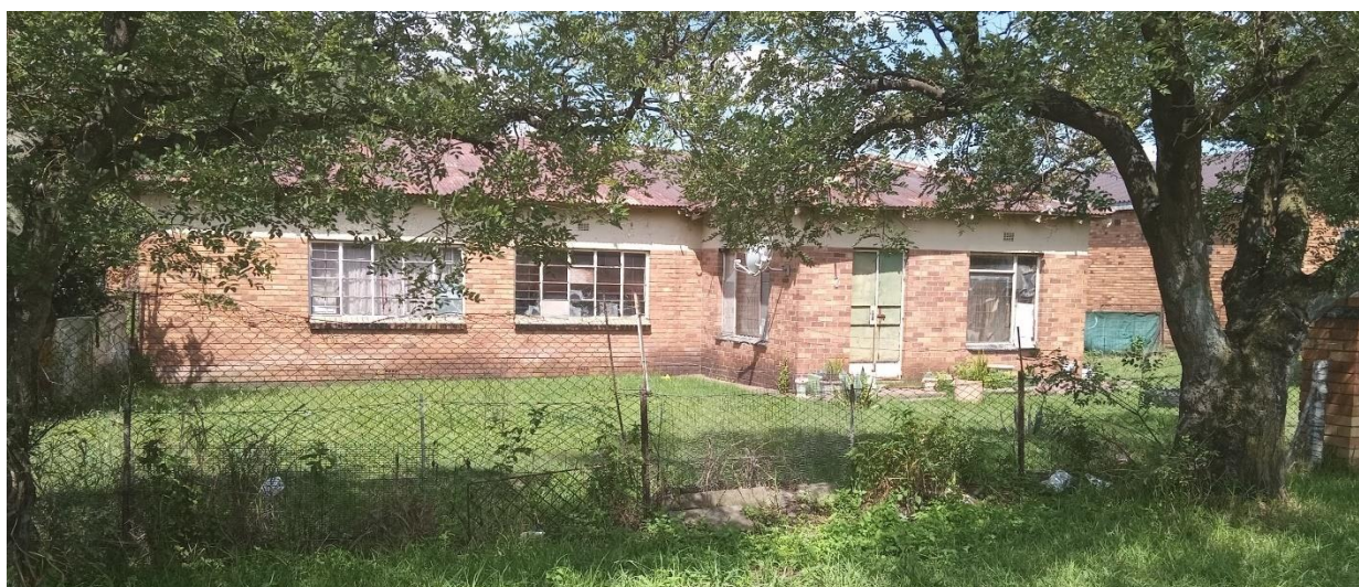
Figure 90:View of the one of the two historical houses at CCUS-27
