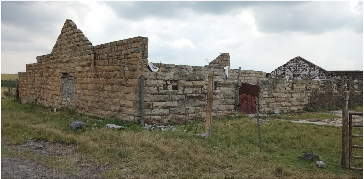
Figure 53: View of the larger building, one section of which is constructed sandstone
