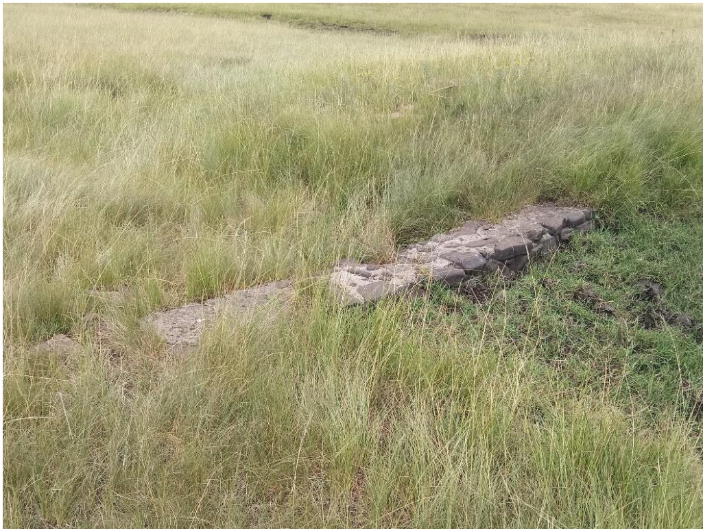
Figure 44: View of the stone dam wall/weir structure
