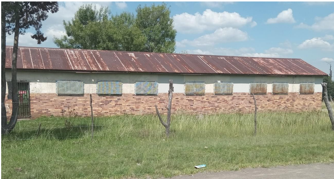
Figure 94: View of the third building
