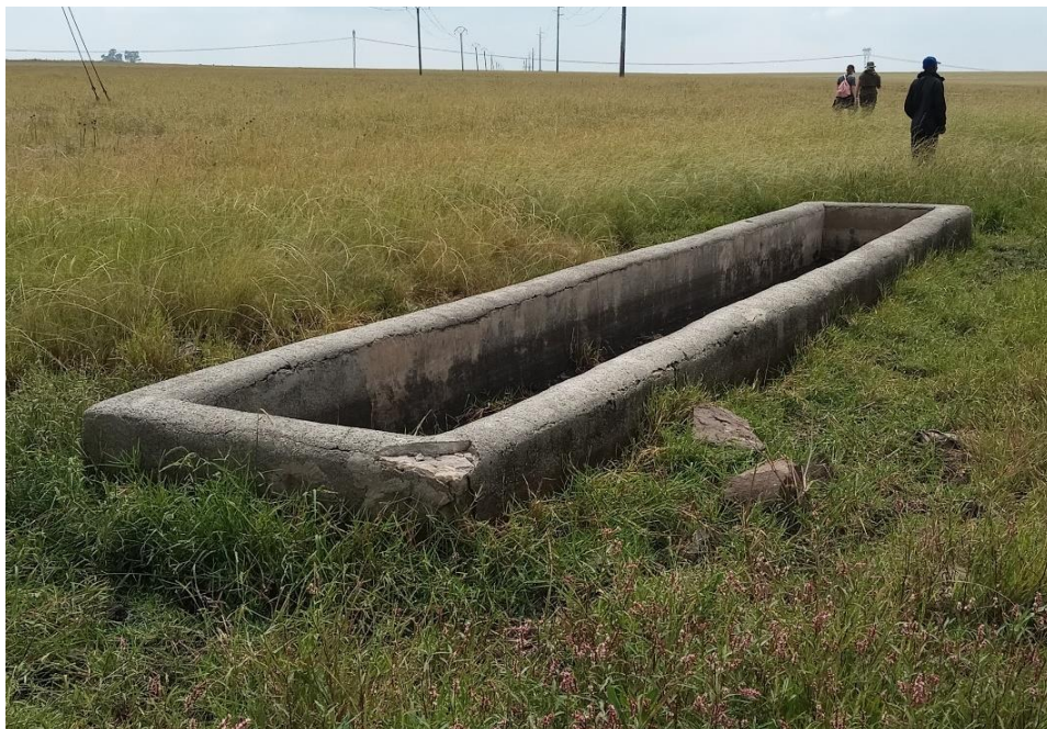
Figure 37: View of large trough, covered in cement
