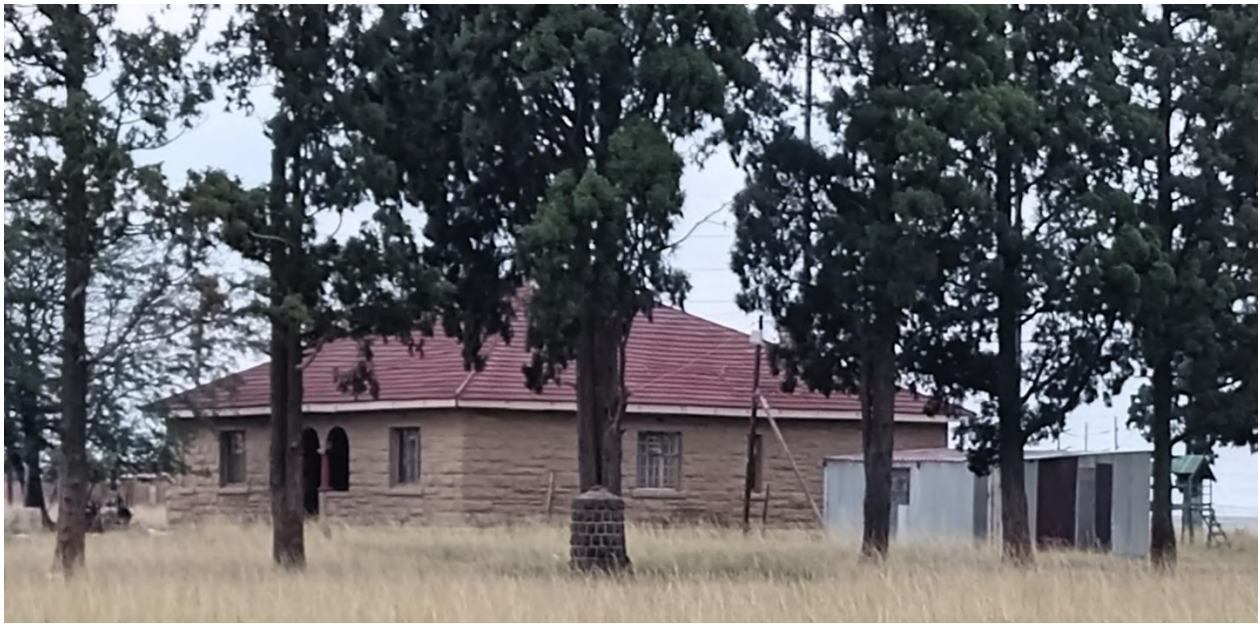
Figure 56: View of the historical sandstone house at CCUS-13, showing the north and west elevations
