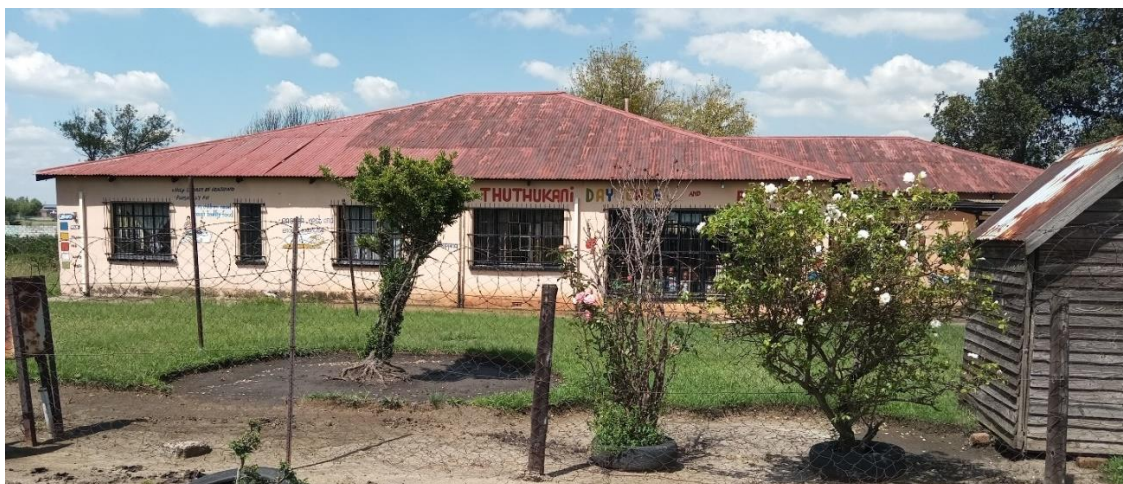
Figure 86: View of house at CCUS-24, taken from the road
