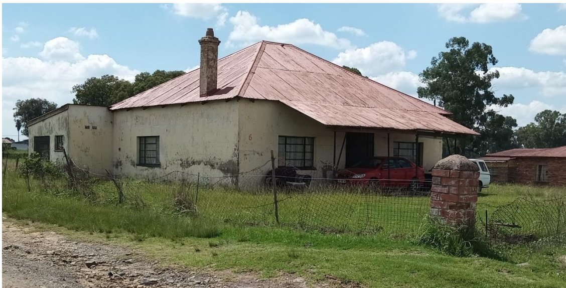
Figure 80: View of historical house at CCUS-22
