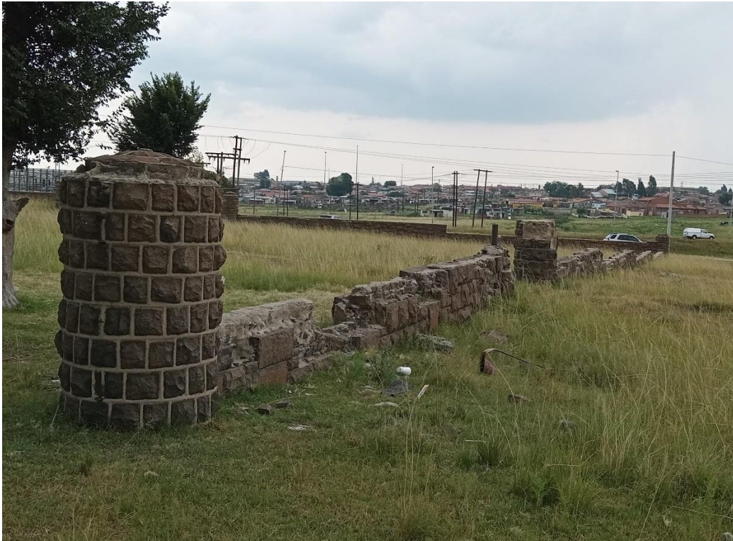
Figure 60: View of the surrounding wall, built from dolerite stone, showing one of the circular pillars
