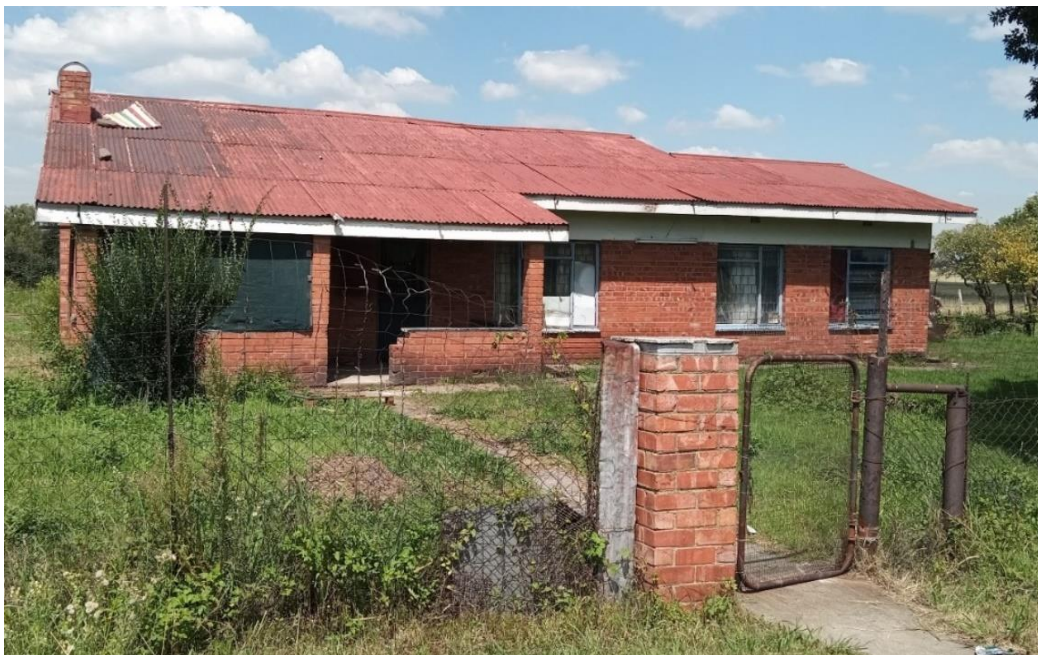
Figure 87: View of historical house at CCUS-25
