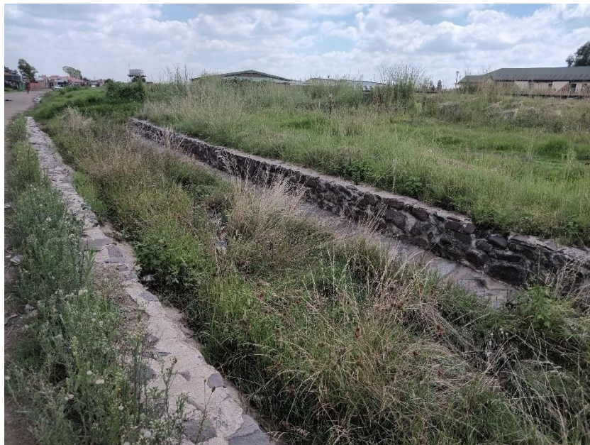
Figure 75: View along the stone water channel at CCUS-18
