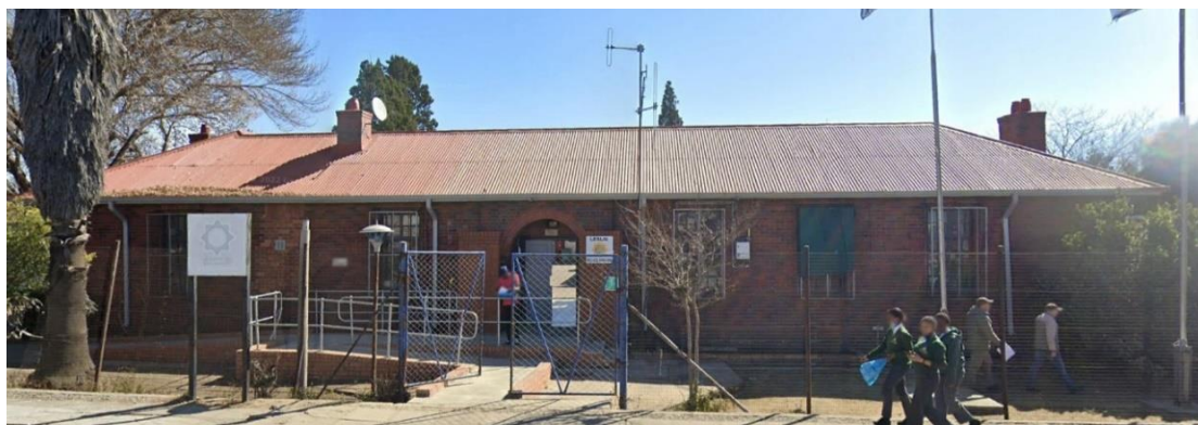
Figure 14: View of historical police station building on north side of Leandra Main Road/R29 (R29 (Google earth Streetview)
