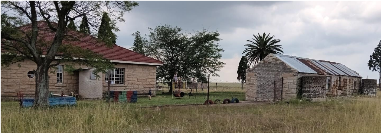
Figure 58: View of the south elevation of the house, showing the sandstone outbuilding on the south side
