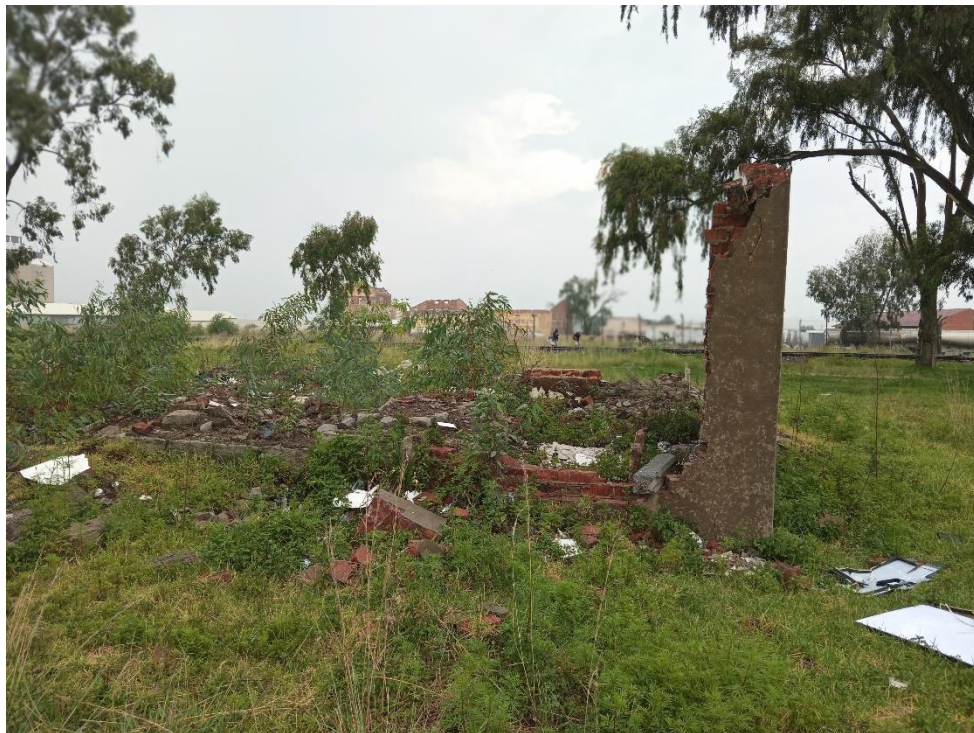
Figure 67: View of another of the demolished houses with a piece of brick wall remaining
