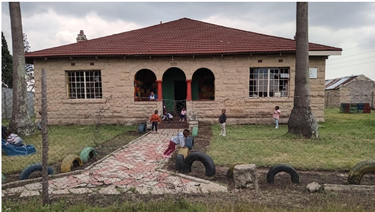
Figure 57: View of the front (west) elevation of the house, note the associated outbuilding visible on the south side.
