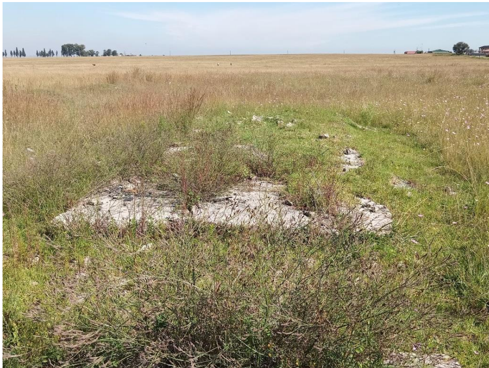
Figure 98: View of the other foundation
