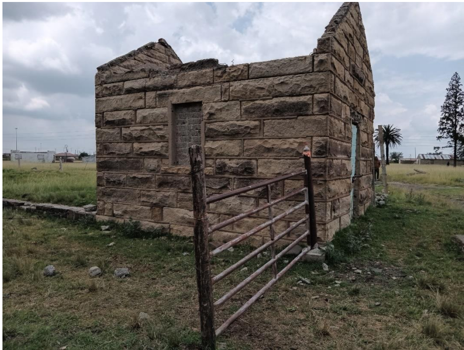
Figure 51: View of the smaller sandstone building
