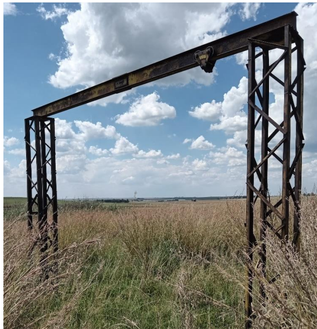
Figure 108: View of metal structure
