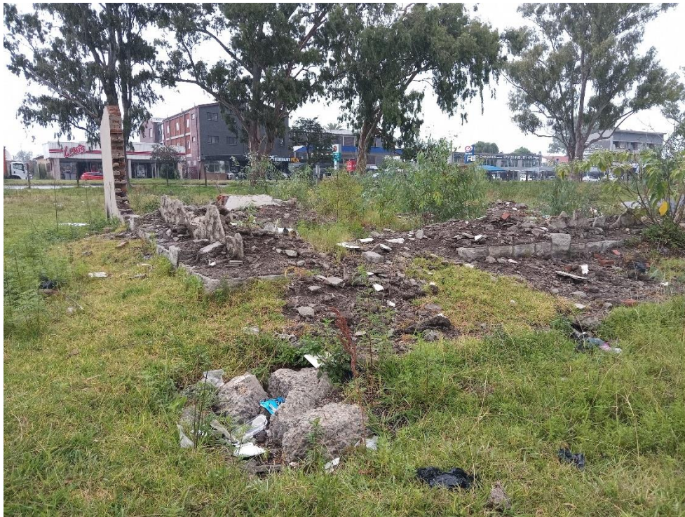
Figure 66: View of the foundation remains of another house with a piece of brick wall surviving
