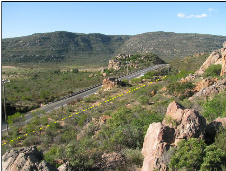
B: PLR 10, the old road (dotted line) can be seen in places and dry stone embankments are quite distinct. No impacts are likely to occur to this feature. The powerline will be in the valley to the left of the road.
