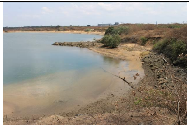
H Excavated harbour edge
