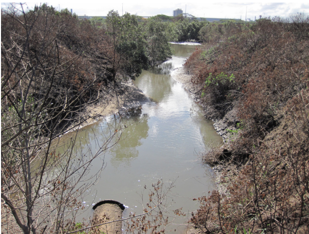
Photo 9: Near high tide at the point of entrance of pipe carrying tidal water into the Shallow Intertidal area at Site C.
