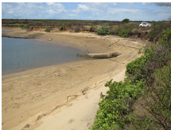
Photo 11: Inlet point of connection pipe in the 'Caisson' basin.
