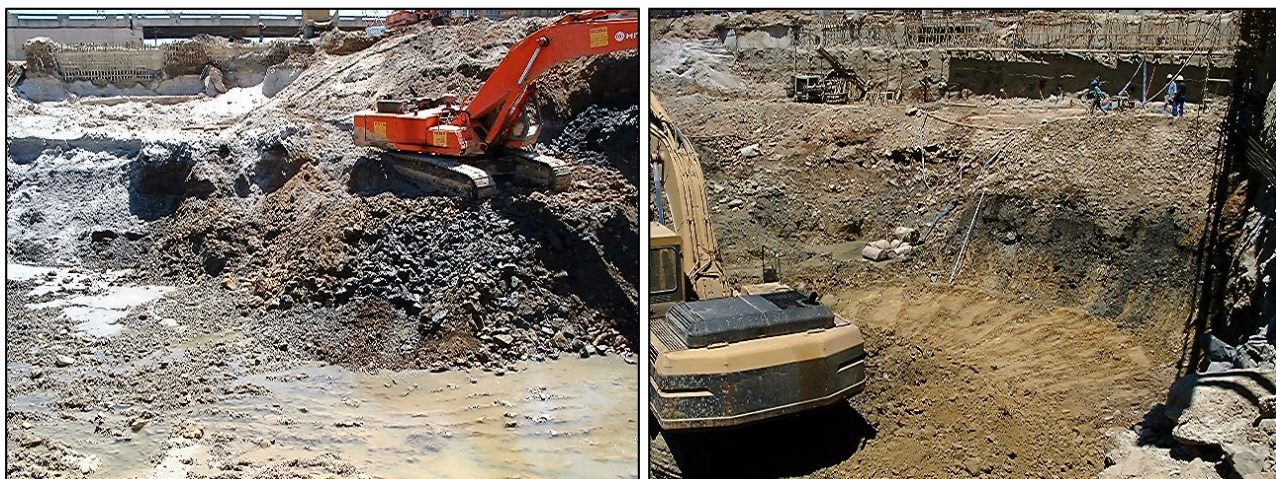
Plates 23 & 24: At left two types of fill consisting of the lower rock rich deposits (from the base of Duncan Dock?) and sea/dune sand above. A thick dark layer in the photograph at right, was interpreted as the old seabed, upon which was a build up of organic debris and coal residue (Photographs: ACO Associates archive).
