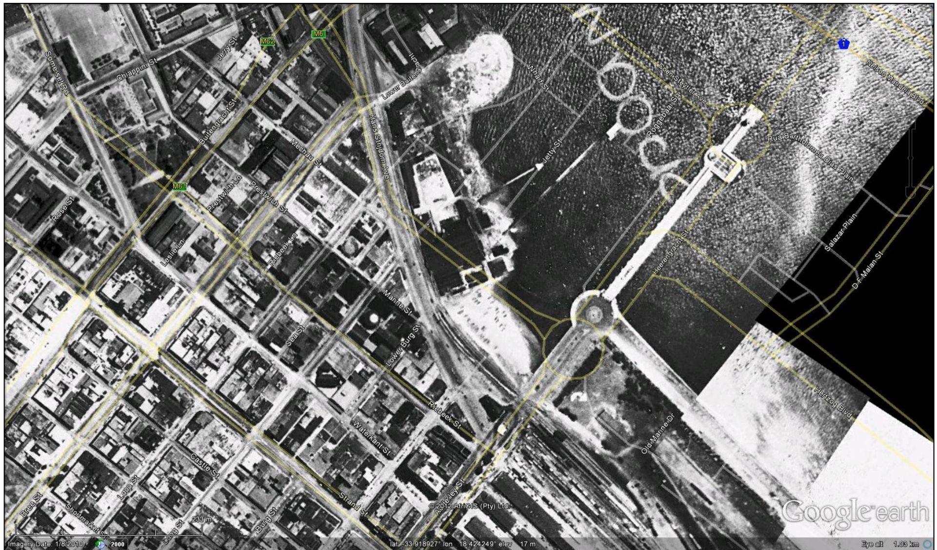
Figure 7: An extract from the 1926 aerial photo of Cape Town showing the 1913 pier (source: Jordan 2003) with current street map superimposed via Google Earth. The old Roggebaai fishing boat harbour and beach clearly visible at center The old promenade running south east from the base of the new pier at the foot of Adderley Street.
