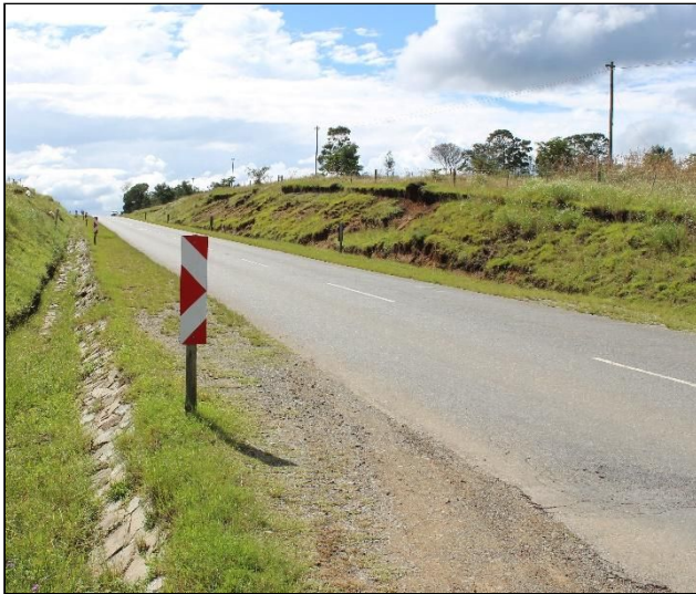
Plate 18: Storm water drainage channels [1]
