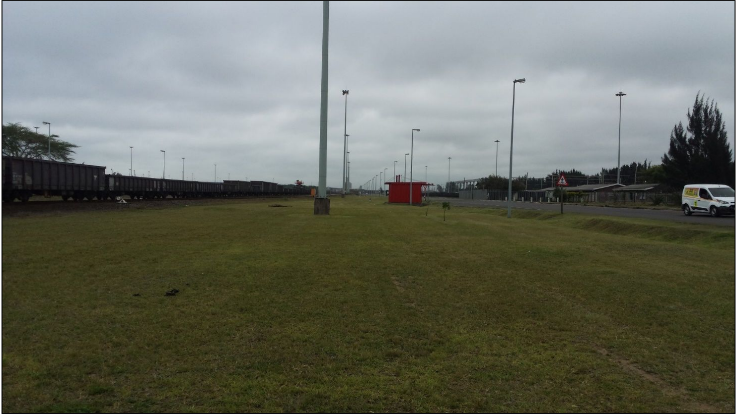
Figure 7.9 Existing infrastructure along pipeline route
