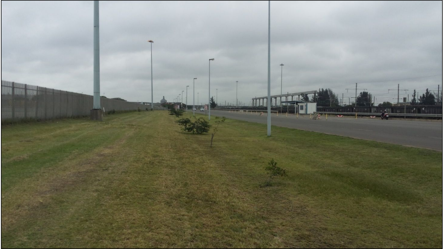
Figure 7.11 Existing infrastructure along pipeline route
