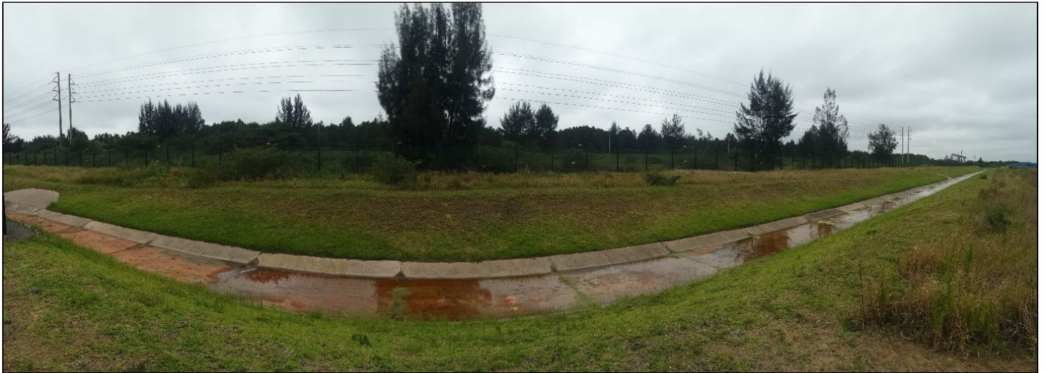
Figure 7.3 V drain channels to drain previous swampland.
