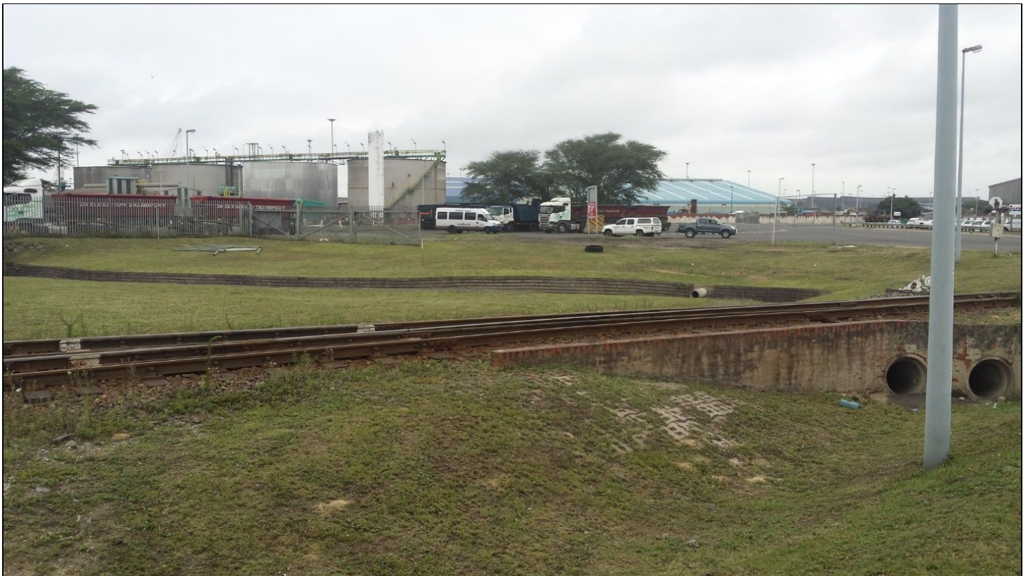
Figure 7.12 Existing infrastructure along pipeline route
