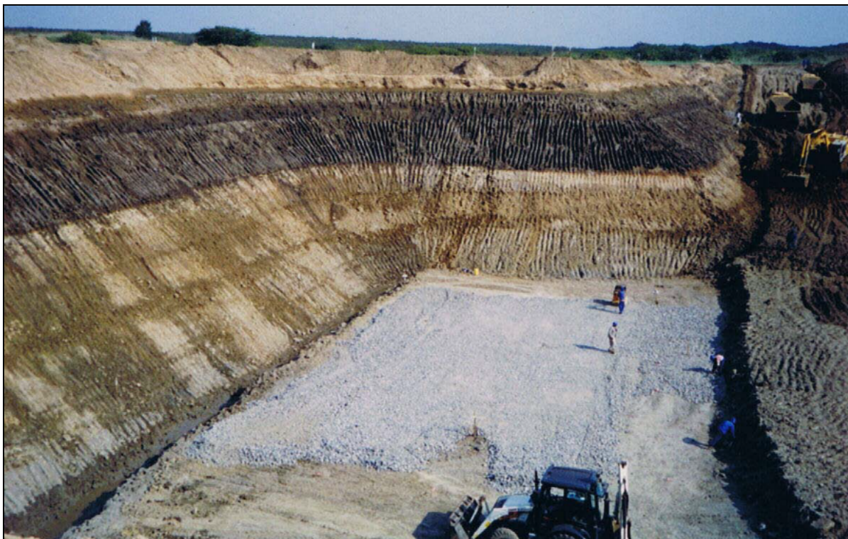
Figure 3. Excavations at Berth 306, Richards Bay Harbour. Exposure of Cretaceous horizons at 14m below m.s.l.
