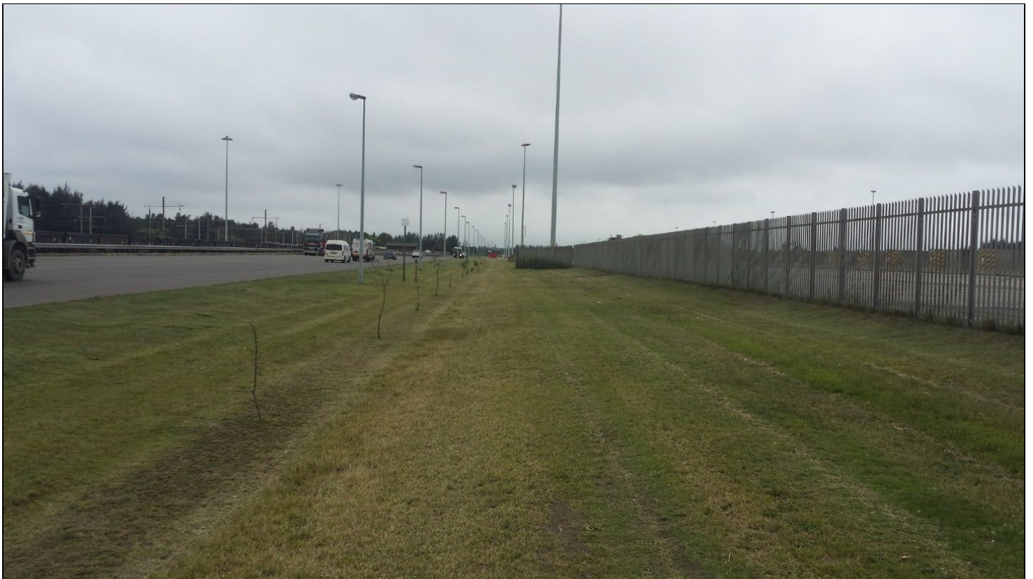
Figure 7.10 Existing infrastructure along pipeline route
