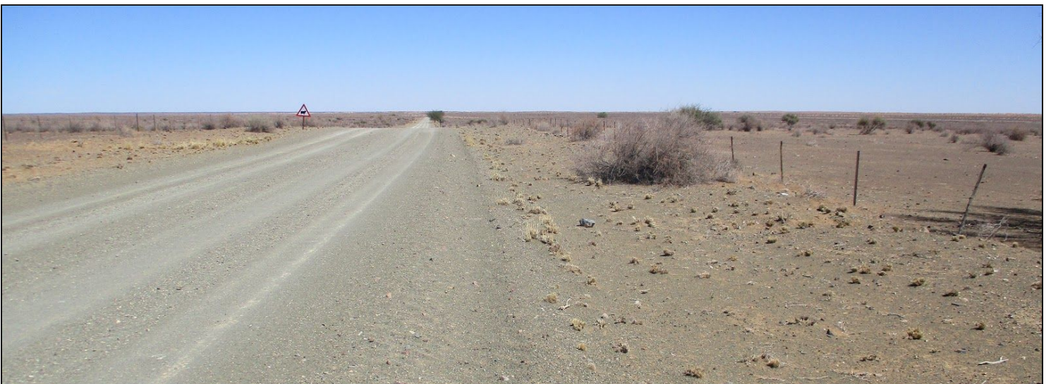
Figure 8.7: Contextual Images: View over proposed pipeline route
